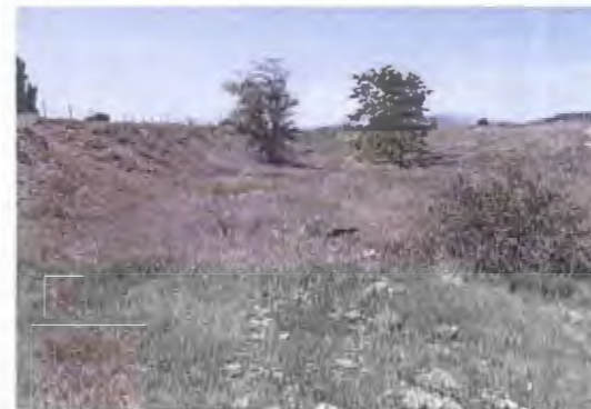
Photo 9. Embankment and concrete piles in Arroyo de las Calabasas
