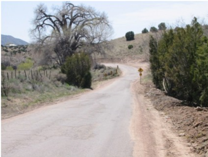
Unpaved road in La Cienega
