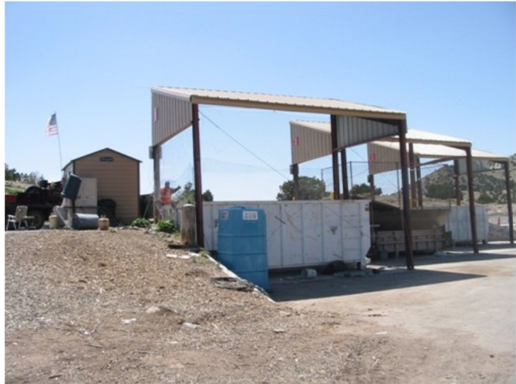
La Cienega Transfer Station at County Road 54B
