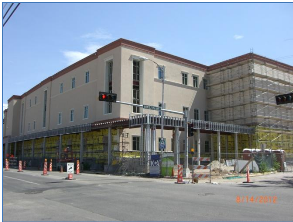
Exterior building looking northeast
