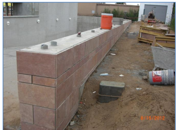
Stone work at site walls
