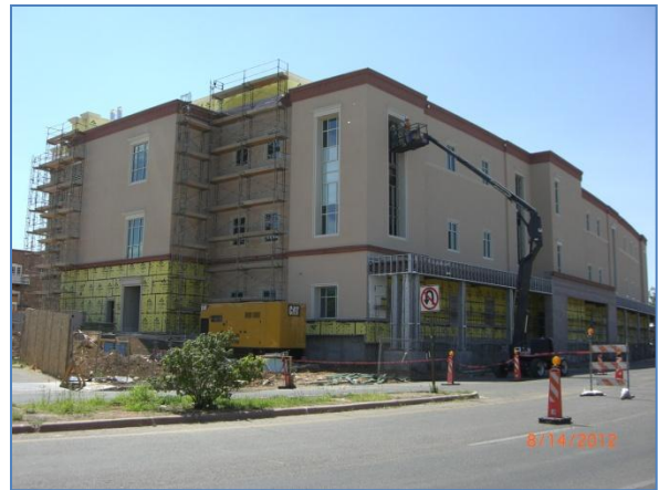
Exterior building looking southeast
