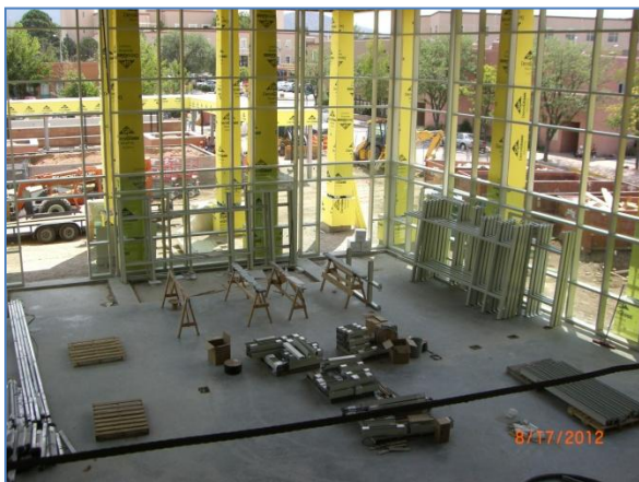
Storefront framing at lobby area
