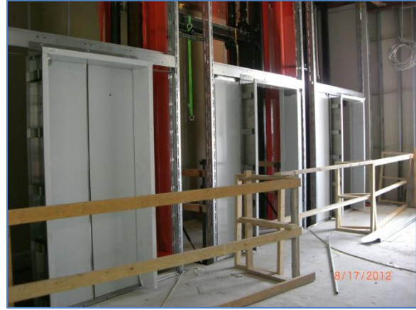
Elevator work on first floor
