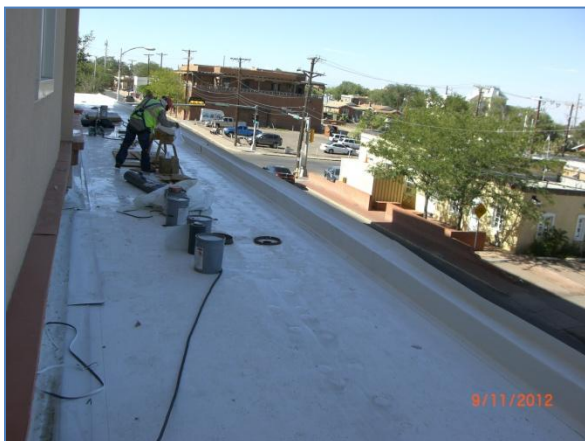
Roofing at west portico
