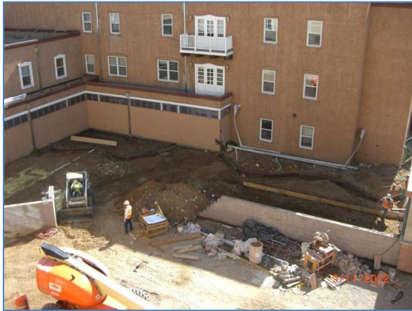
Sitework at DA courtyard
