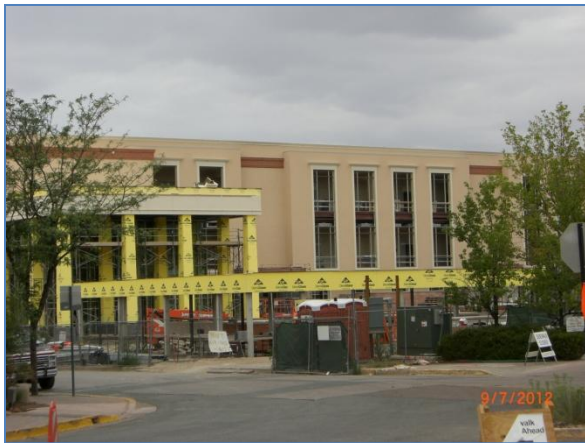
Exterior building looking west
