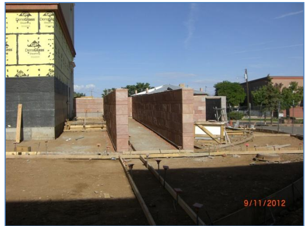
Handicap ramp at north end of building
