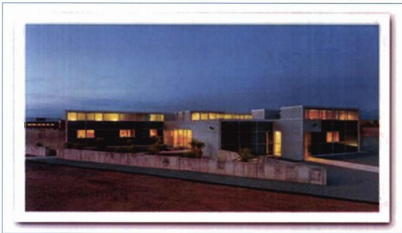
Santa Fe County Public Works Facility
