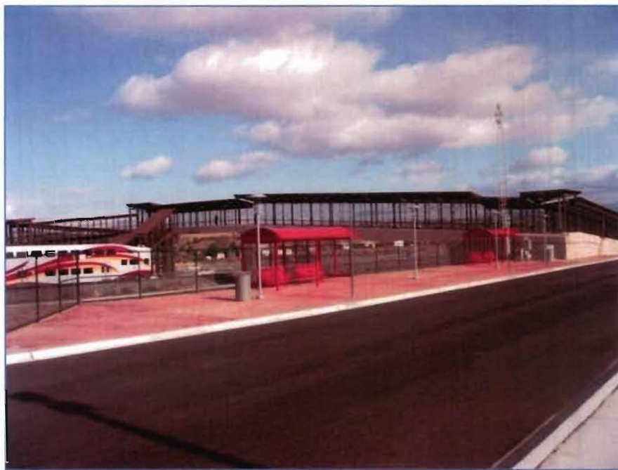
Rail Runner Station at NM 599
