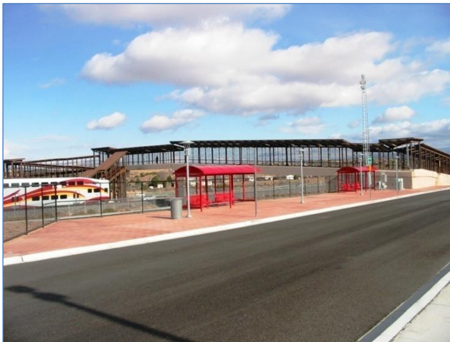
Rail Runner Station at NM 599
