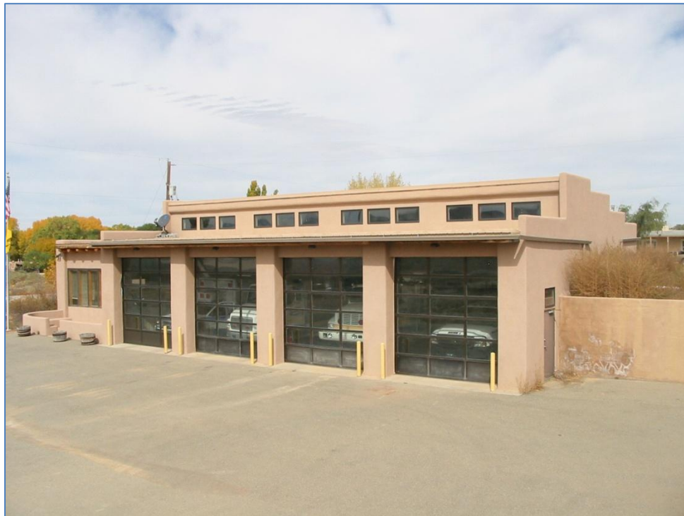
Galisteo Fire Station
