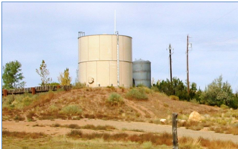
Galisteo Water Tank
