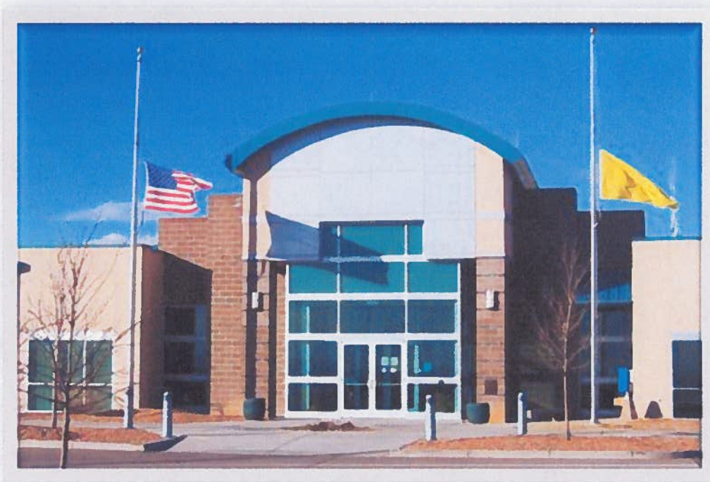
Santa Fe County Public Safety Complex
