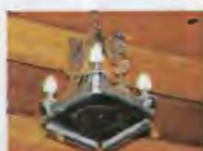
One of the hammered-and-pierced tin light fixtures in conference room
