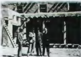
Left to Right: Charles Gable, Herb Maier, Tom Bales & Hugh Miller watch progress on the new headquarters
