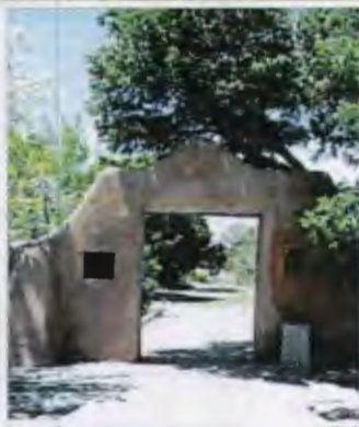
Entrance gate flanked by CCC and National Historic Landmark and bronze plaques
