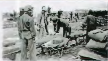
CCC workers laying adobe bricks, 1938
