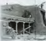
Building under construction, 1938
