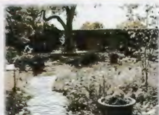
The Old Santa Fe Trail Building has not changed significantly in character or use since its completion in 1939
