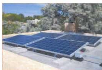
Ballasted (weighted) PV system.
