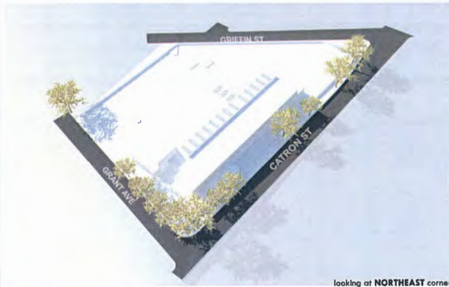
looking at NORTHEAST corner
