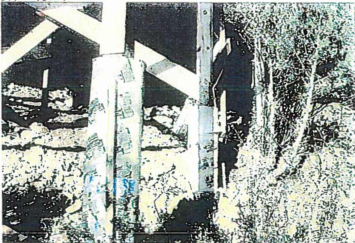
OPTIONAL RETAINING WALL WOULD PREVENT SOIL EROSION AROUND CONCRETE BASE SECTIONS, HOWEVER - NO EVIDENCE OF EROSION HAS BEEN DETECTED FOLLOWING HARD RAINFALL SEPT 20. THEREFORE RETAINING WALL IS LIKELY NOT NECESSARY. WILL ADD OR OMIT WALL AS PER PANEL RECOMMENDATION.
