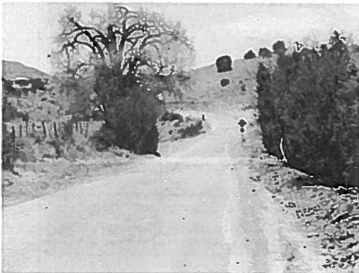
Unpaved road in La Cienega
