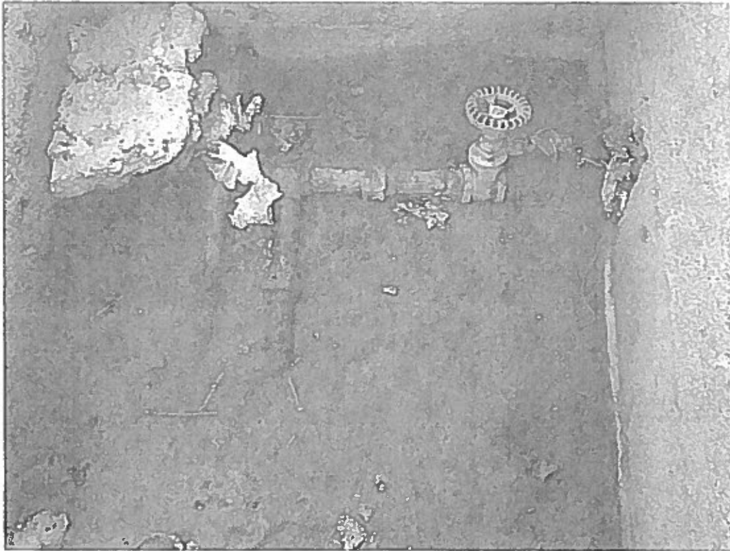
Figure 17: Station 294+38 valve junction box for water diversion to La Bajada storage tank. Photo by field team, spring 2011.
