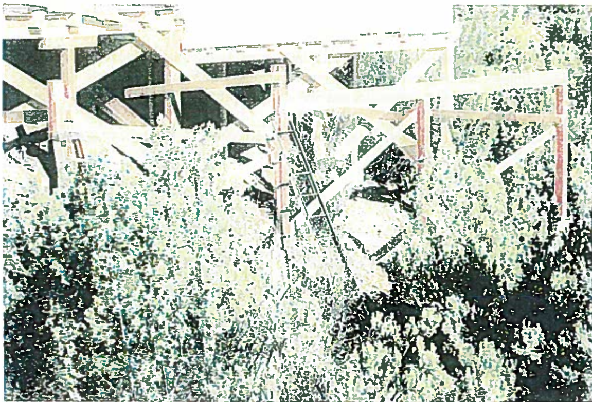
CONCRETE + POST CONSTRUCTION ON SLOPE WITH CROSS BRACING LADDERS SHOWN LEANING AGAINST POSTS FOR DECK (SOUTH SIDE) TO ADD STRUCTURAL INTEGRITY - WIDER FOOTPRINT WITH VERY LITTLE ADDED WEIGHT
