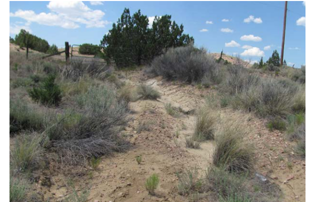
Eroded access road to EAWSD well.
