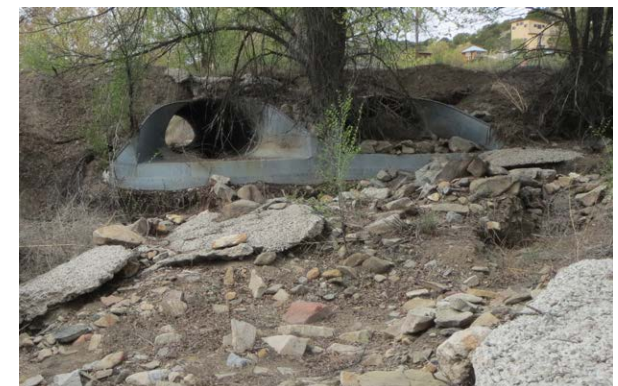
Culverts at Cave Rd. crossing, right-hand culvert clogged.
