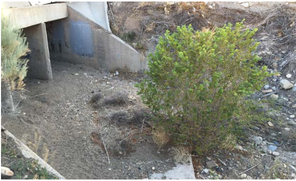
Trees growing in active channel impede flood flows.
