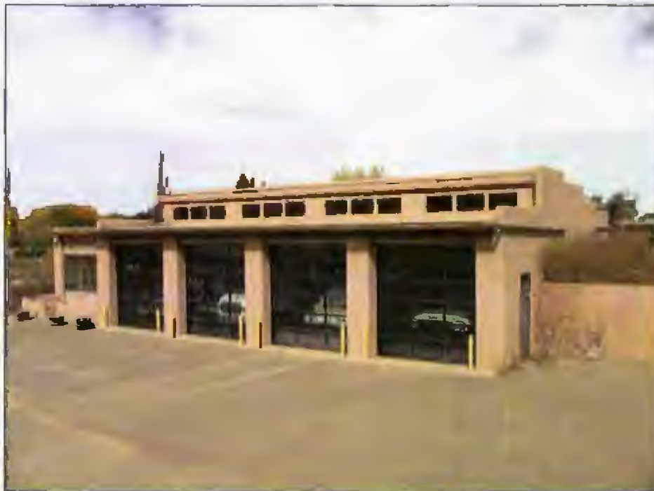
Galisteo Fire Station
