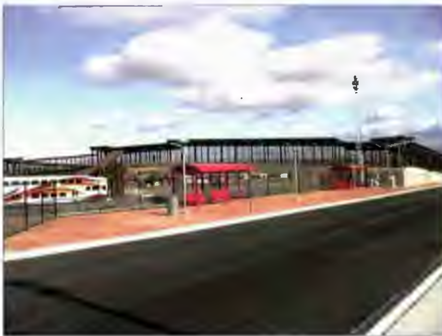
Rail Runner Station at NM 599
