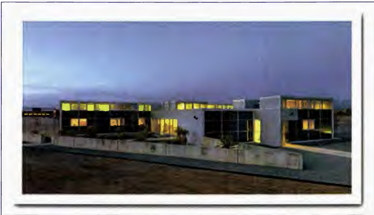
Santa Fe County Public Works Facility
