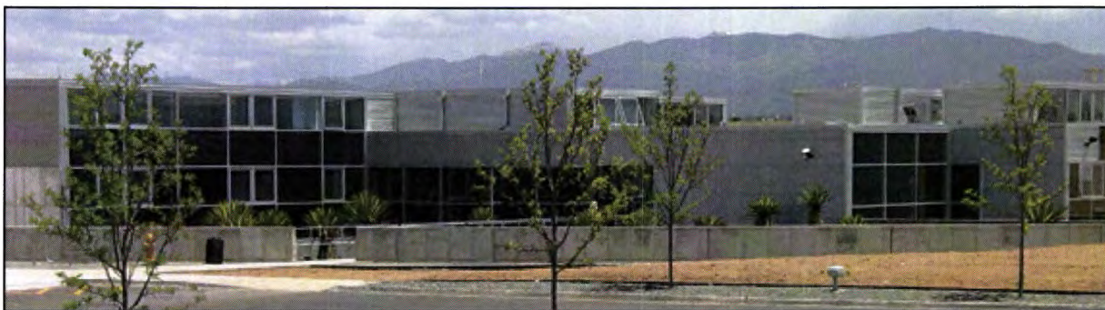
Santa Fe County Public Works Complex. Santa Fe, NM
