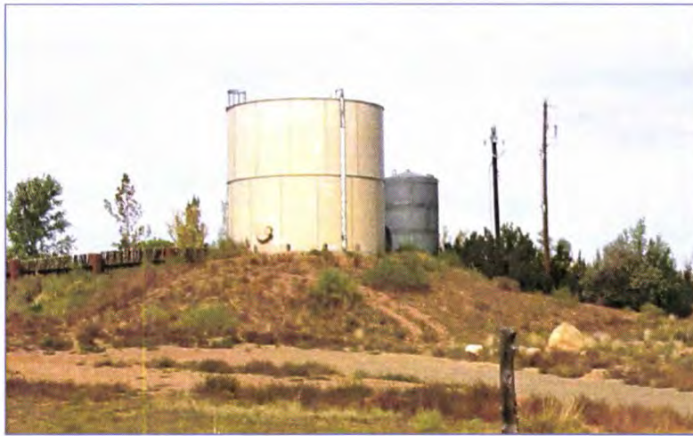
Galisteo Water Tank
