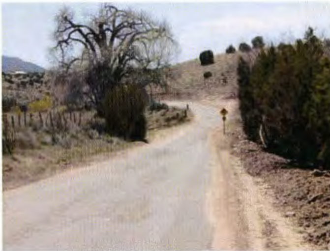
Unpaved road in La Cienega
