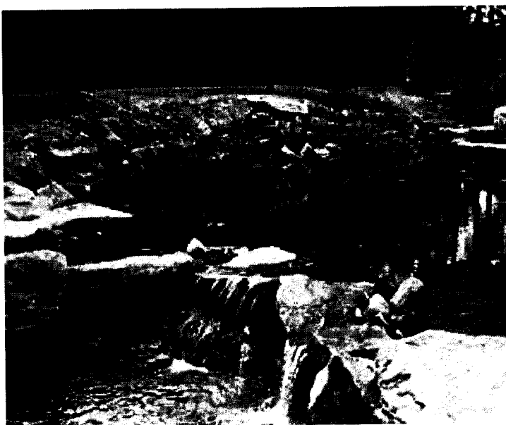
Figure 24. Image of a rock vane centering the flow. Source: Conejos Canyon Ranch.
