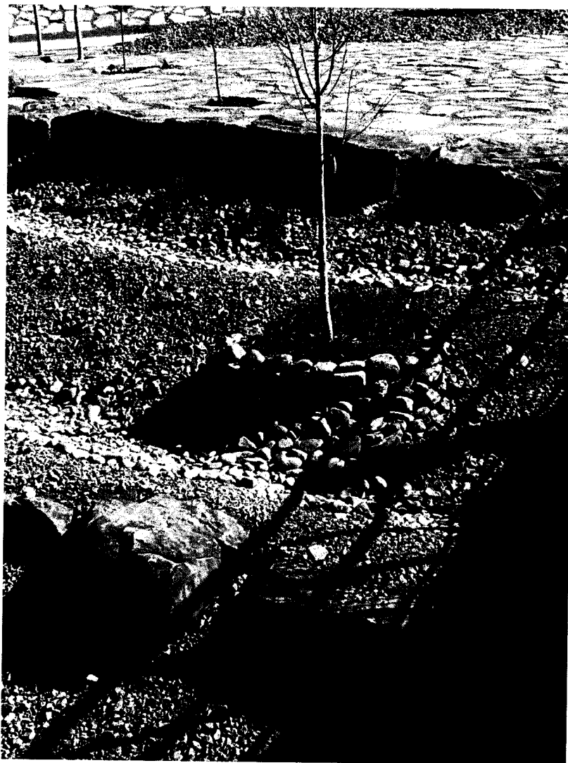
Figure 46. Image of an individual tree terrace with a rock retention wall. Source: Ecotone Landscape Planning 2018.
