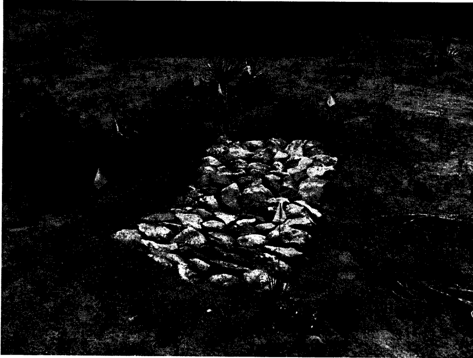
Figure 33. One-rock dam in upland areas. Photo: Ecotone Landscape Planning.
