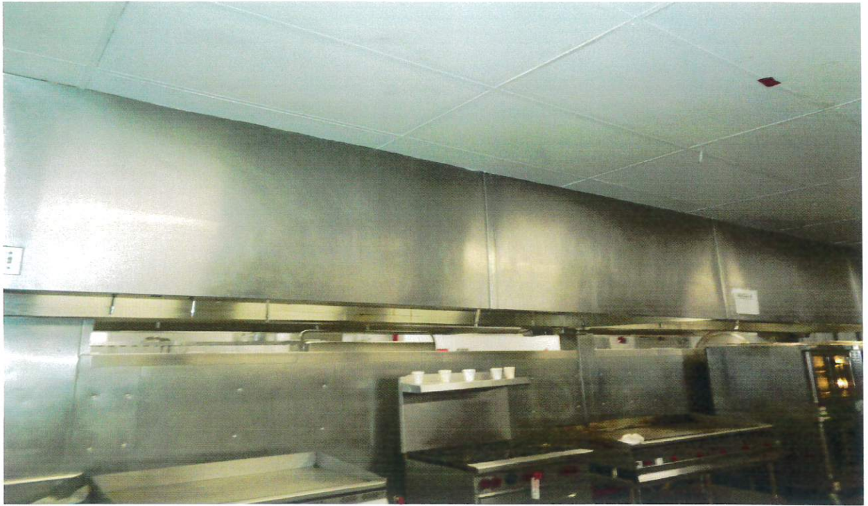
Exhaust fan/ ports with extinguisher system
