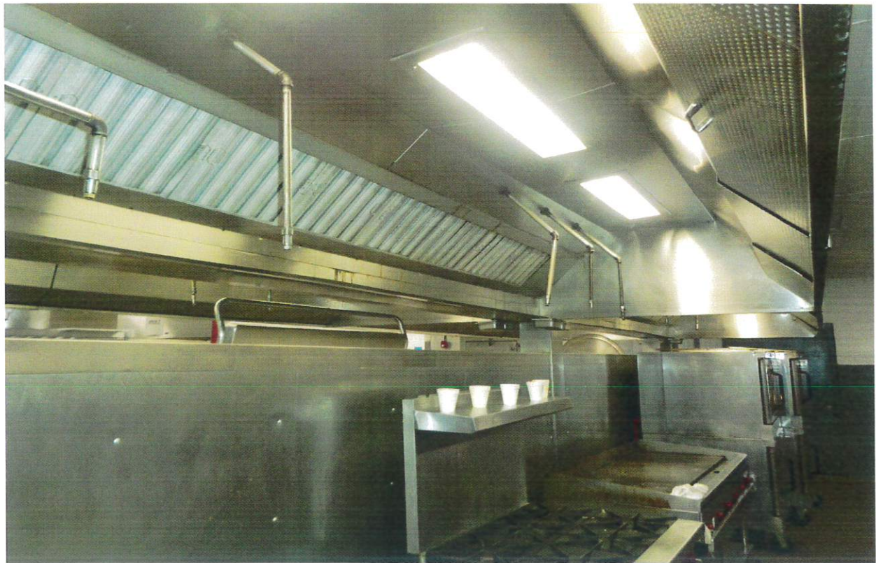
Exhaust fan/ ports with extinguisher system
