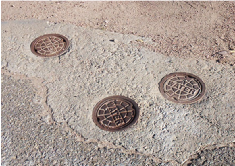
Photo 9: Water Main/Lateral Isolation Valves
