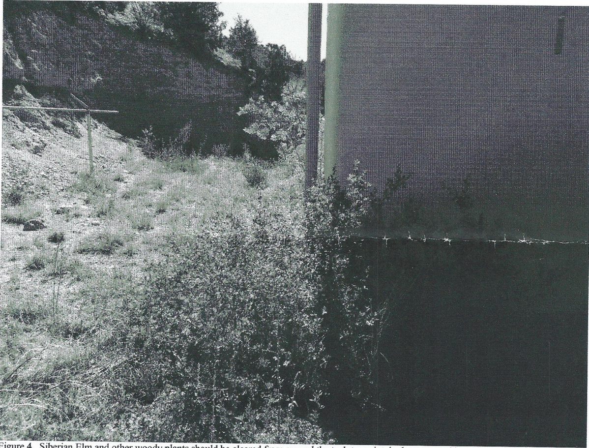
Figure 4. Siberian Elm and other woody plants should be cleared from around the tank to maintain the structural integrity of the facility.
