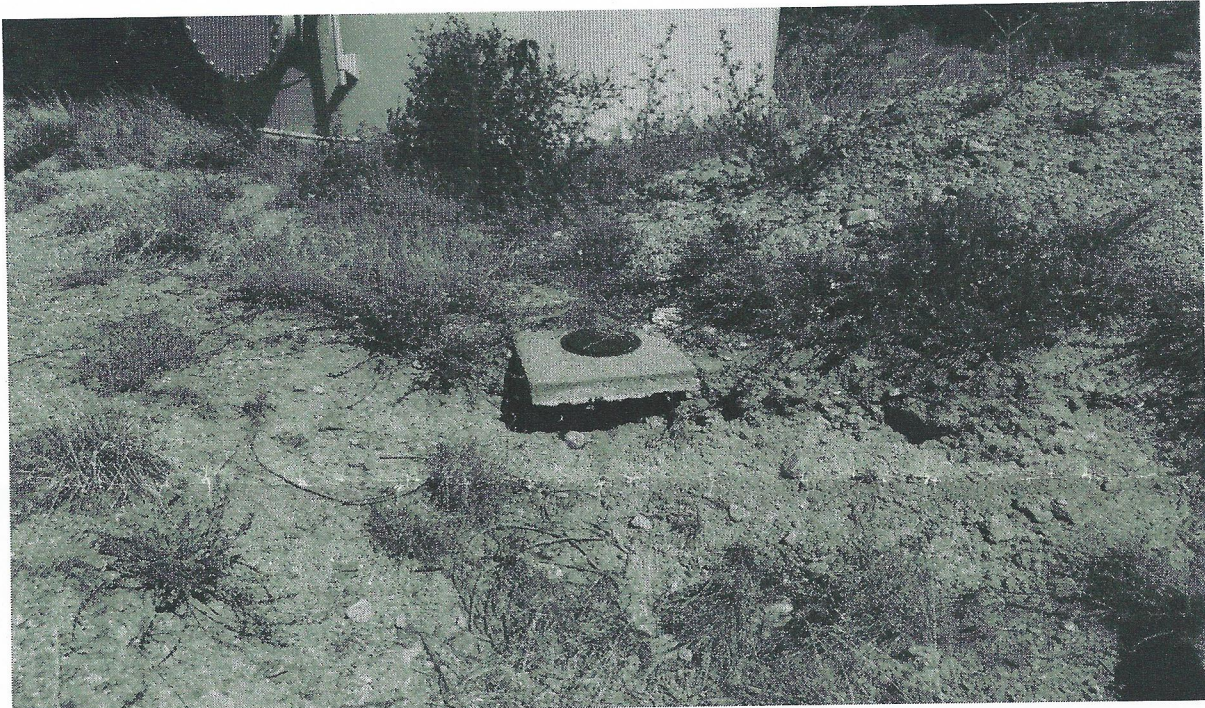
Figure 1. Significant Deficiency #2. Erosion near storage tank facility.
