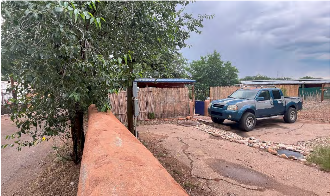
Frame 9. HCPI 54937, Front (southwest) elevation showing property boundary wall. Camera View Northeast.
