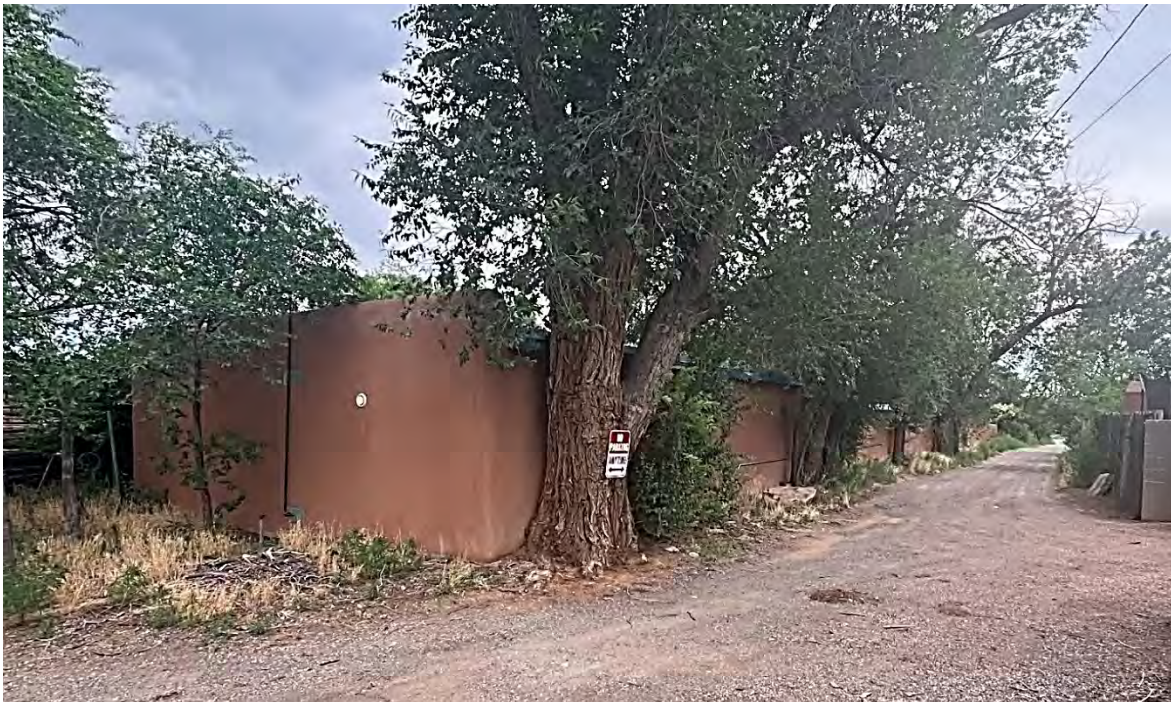
Frame 6. HCPI 54937, Northwest (side) and northeast (rear) elevations from project area. Camera View Southwest.
