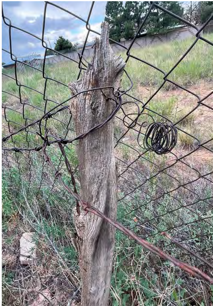
Frame 11. IO 5. Fence post with barbed wire adjacent to contemporary chain-link fence.
