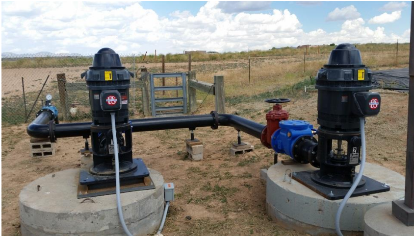
Figure 6: Existing Reuse Irrigation Pumps
