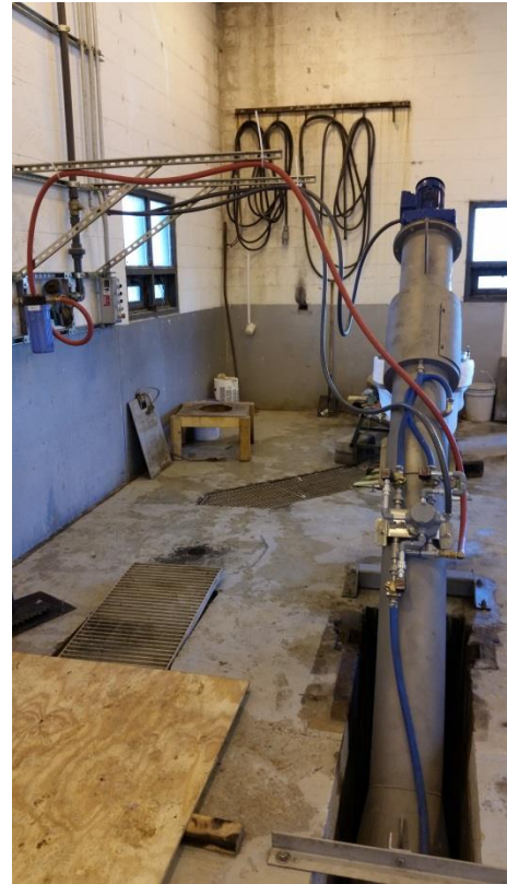
Figure 4: Existing 6 mm Lakeside Screen
