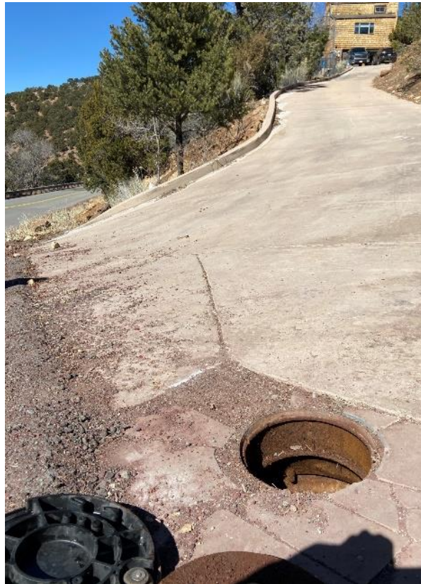
Photo 6 – Existing Meter Vault Example in HPE
