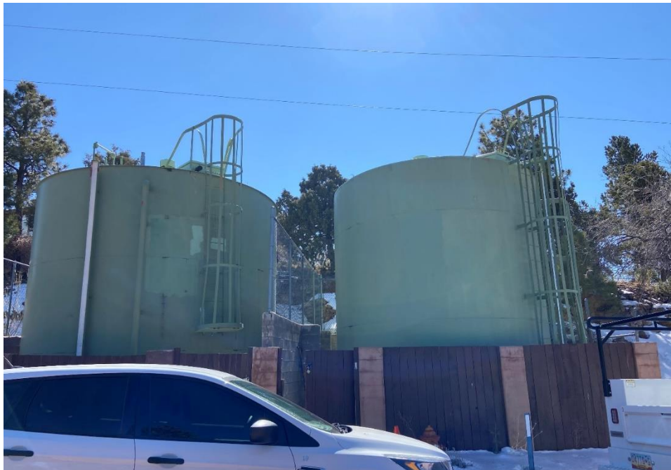
Photo 3 – Existing Water Storage Tanks
