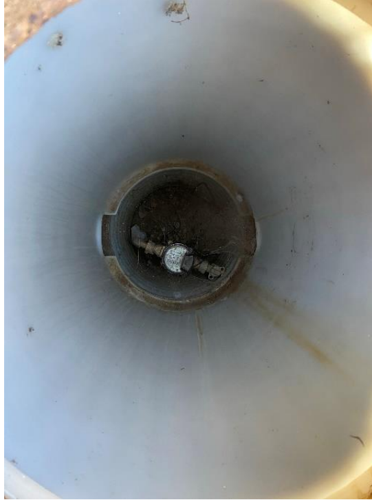
Photo 7 – Existing Meter Vault Example in HPE
