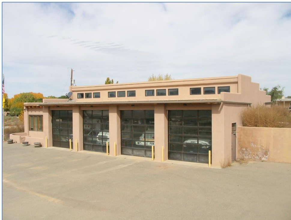
Galisteo Fire Station
