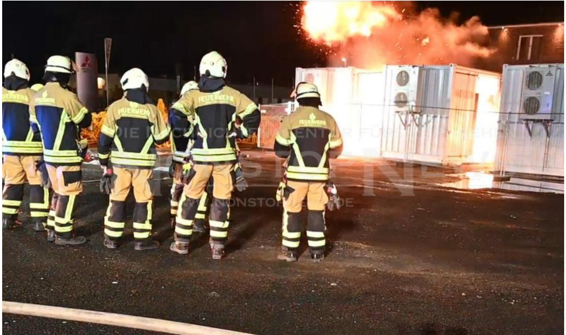
Fire at Neermoor, Germany Battery Storage Site
