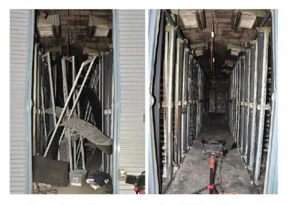
Interior damage to the BESS after the explosion [left], and after debris was removed to gain access to begin the forensics analysis [right].
