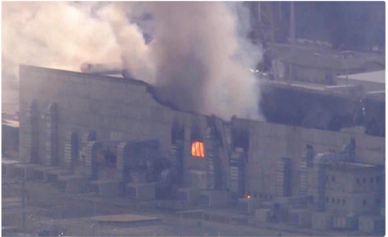
Figure 5 – Moss Landing Lithium Battery Facility Fire 7
