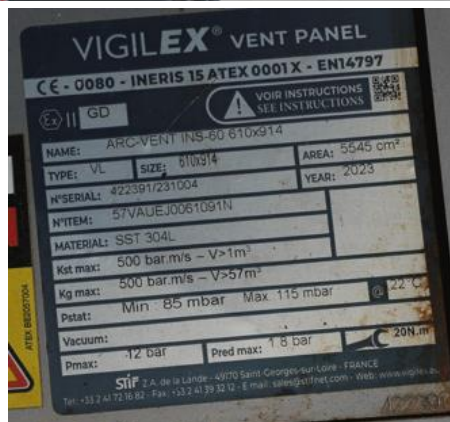
Figure 2.5: Location and specification of deflagration panels on top of container
