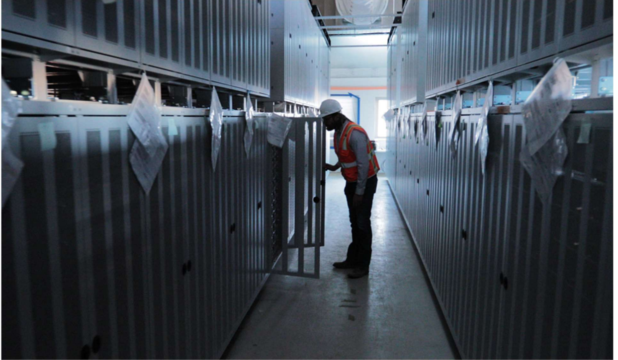
5 Figure 1: Indoor Battery Packs at Moss Landing BESS 4
