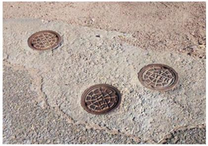
Photograph 10: Water Main/Lateral Isolation Valves
