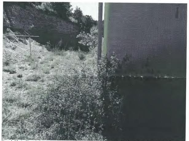
Figure 4. Siberian Elm and other woody plants should be cleared from around the tank to maintain the structural integrity of the facility.
