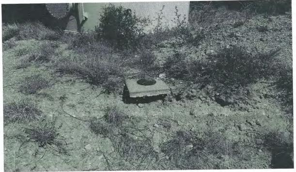
Figure 1. Significant Deficiency #2. Erosion near storage tank facility.
