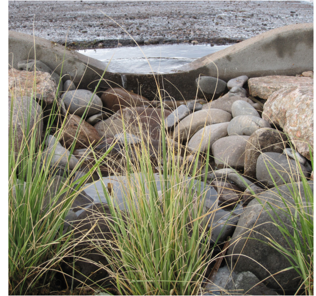
Figure 14. Curb cores (left) maintain the integrity of a curb, but are more prone to plugging with sediment and therefore not generally recommended. Flush curbs (middle) can maximize inflow, but fail to concentrate sediment at a point where it can be managed. Flush curbs might also necessitate the introduction of boulders or vertical core-filled metal pipes to prevent vehicles from damaging vegetation/soil. Moderate (18-24 inches wide) curb openings (right) are ideal for concentrating catchment at a defined point where sediment traps can be installed.
