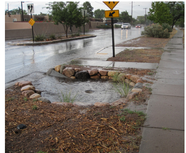
Figure 15. The width of a stormwater inlet for comparable areas of runoff might vary depending on the direction of flow at the capture point. If stormwater is running perpendicular to flow (left), then a smaller opening might suffice. If stormwater is running parallel to the inlet and must make a 90 degree turn into the basin from a small area of runoff (middle), then the inlet width could be improved with a small deflector. As the area of runoff increases, if stormwater is running parallel to the inlet, then a much wider inlet with steeper slope might be required (right). Note that during high intensity storms, runoff in the photo to the right can still bypass the inlet due to originating from approximately 20,000sqft of asphalt area.
