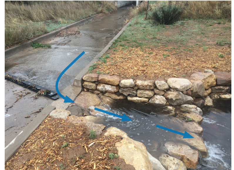
Curb Cut Inlet with Deflector.
