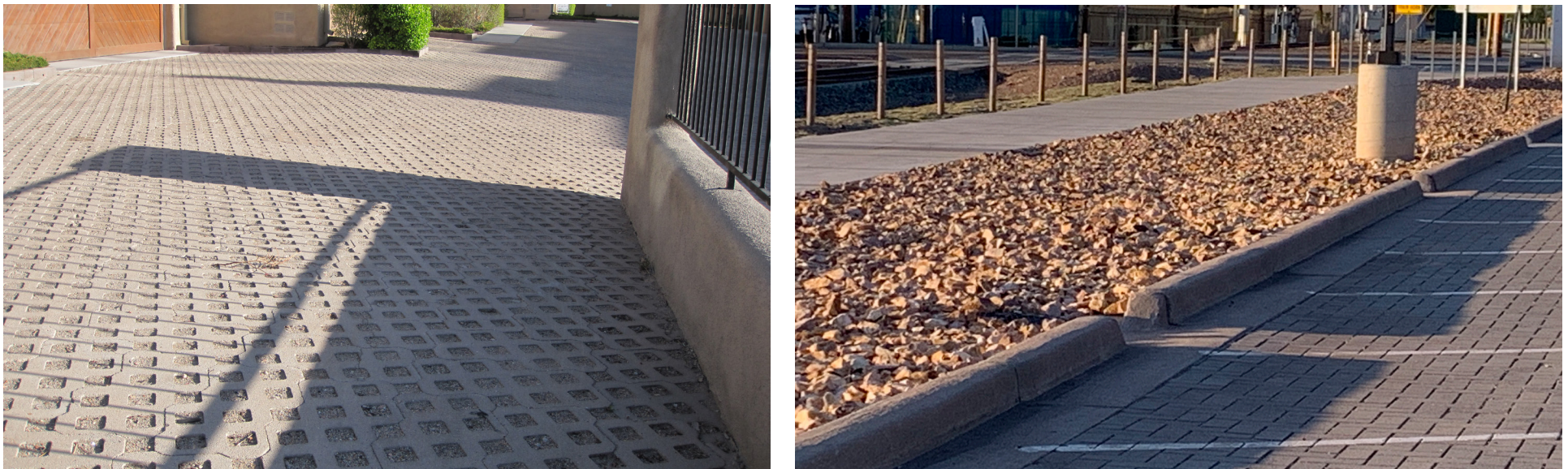
Figure 10. Example of concrete grid paver driveway with minimal sediment sources (left) and permeable interlocking pavers with curb cuts (right) which could direct excess stormwater into other GSI features such as rain gardens (not shown).
