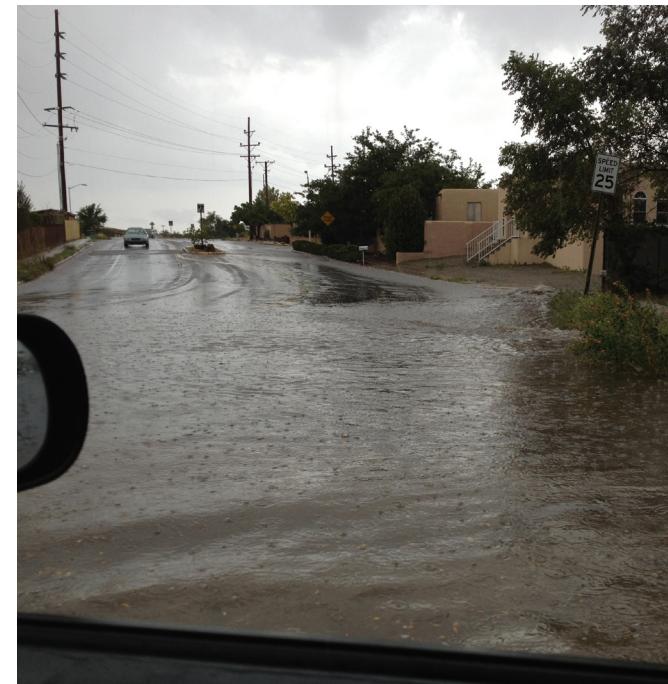
Major storm event causing flooding in street due to lack of appropriate GSI.
