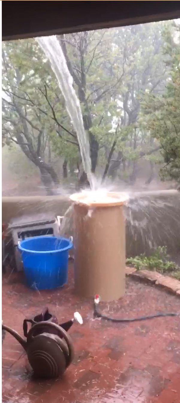
Major storm event overwhelming a rain barrel from roof runoff.
