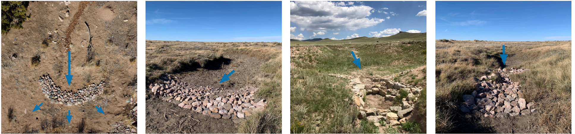
Figure 6. Left to right: A media luna (photo courtesy of Minesh Bacrania), one rock dam, Zuni bowl, and rock rundown are structures used to mitigate stormwater runoff and erosion at low energy upland sites.
