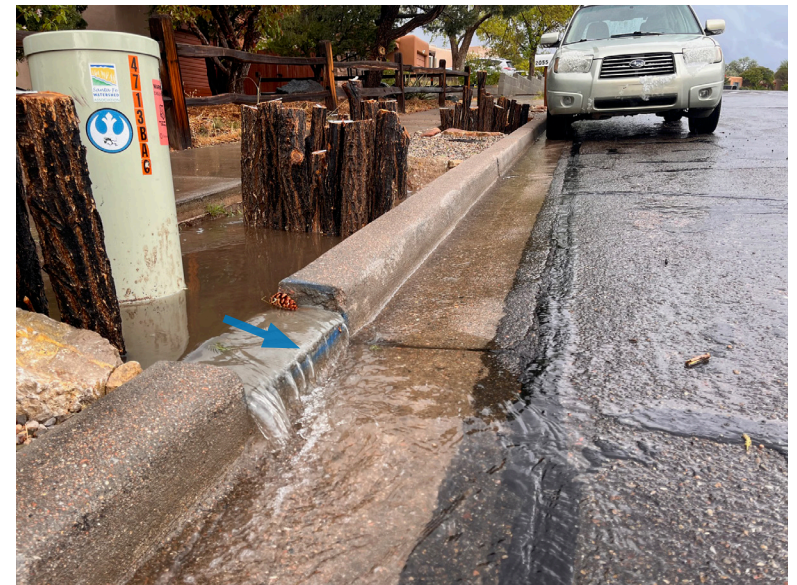
Curb cut outlet at lowest point.
