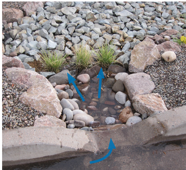
Figure 18. Examples of flow (blue arrows) into sediment traps, and approximate pooling depths before overflow into basins. Left: A small sediment trap approximately 6sqft and five inches deep will capture soil, trash, and other materials from the adjacent parking spaces. Middle: Stormwater runoff from a street is drawn into a sediment trap with a pipe overflow slightly below the elevation of the gutter. Runoff will slow, pool, and drop sediment around the pipe before stormwater overflows into the pipe and passes under the sidewalk into a bioretention basin. Right: A sediment trap in a parking space retrofitted as a rain garden. Bunch grasses in the trap help dissuade pedestrians from stepping into the area when turbid water obscures the depth. Note that while the trap on the right has a smaller volume than the middle trap, the area of runoff is \sim 1/6 the size meaning that the frequency of maintenance could be less.
