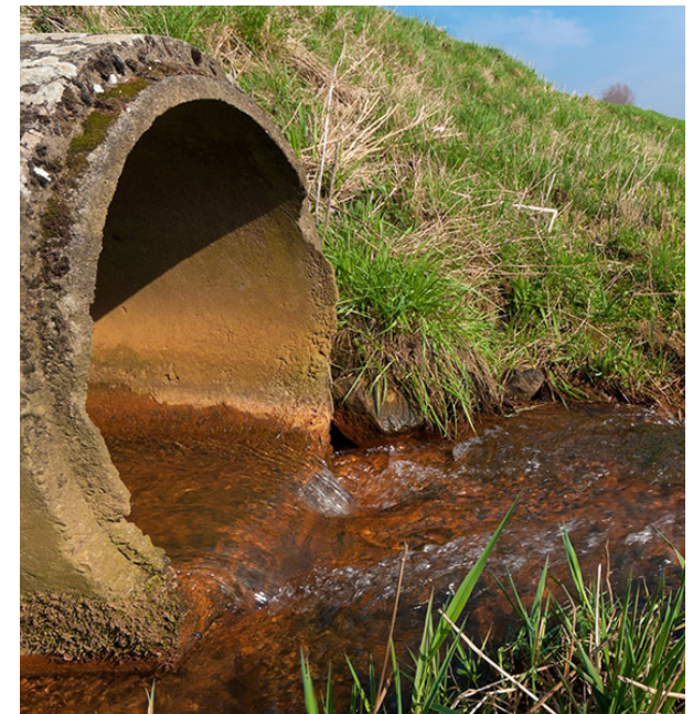
Unfiltered pollutants entering landscape from stormwater outlet.
