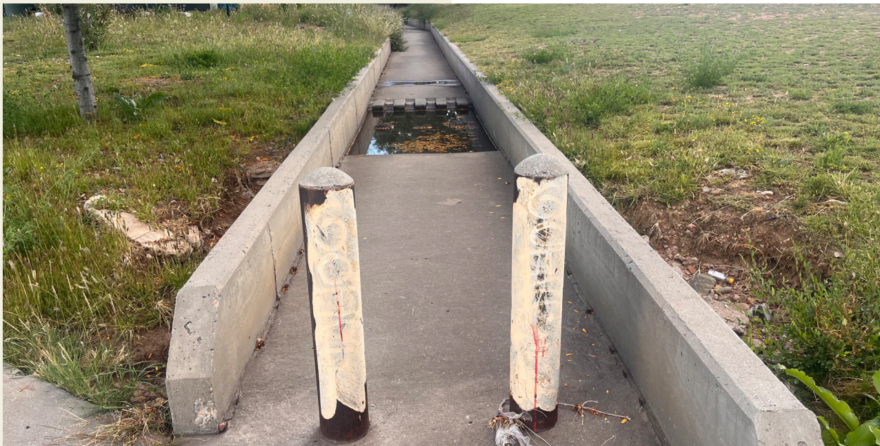
Storm drain cap in concrete channel.
