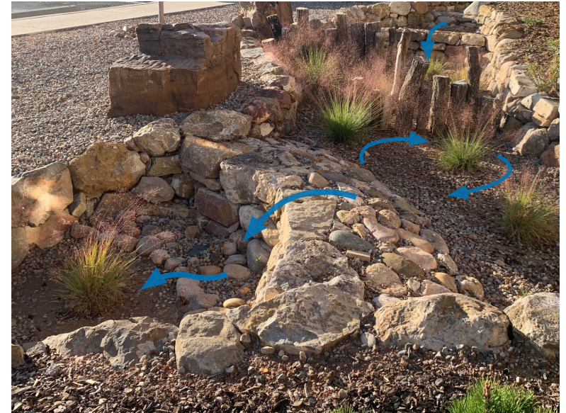
Stone weir construction.
