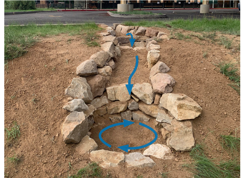
Zuni Bowl Under Construction.
