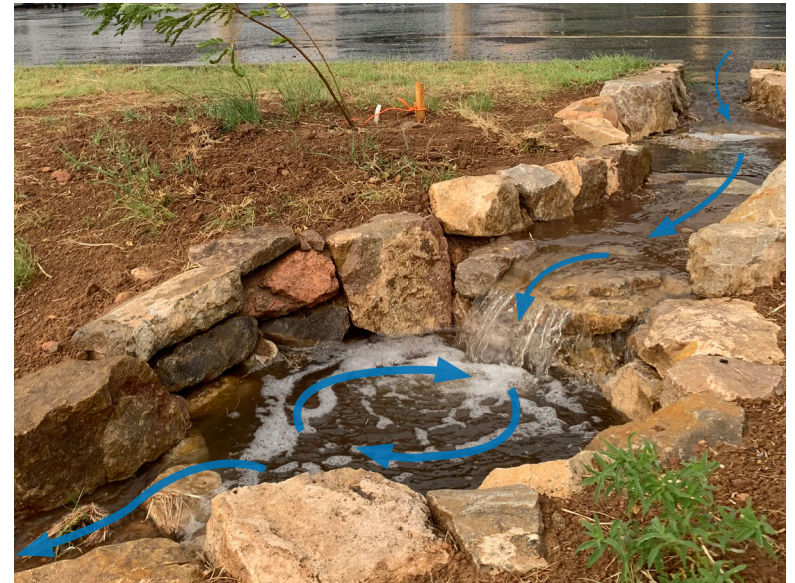
Zuni Bowl Slowing and Stepping Stormwater Down-Slope from Impervious Parking Lot Surface.
