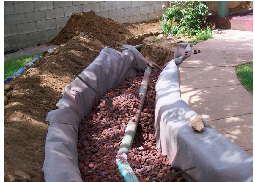
Pumice Wick Trench, Filled.
