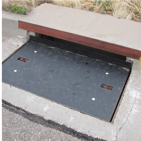
Figure 12. Covering a drain can help “daylight” stormwater so that it continues to flow above ground (instead of a darkened, below ground pipe) to a point of catchment. An estimate of increased discharge should be considered before installing a drain cap to ensure that daylighted runoff will not cause flooding, erosion, or other problems prior to reaching a GSI feature where stormwater is intended to be captured.
