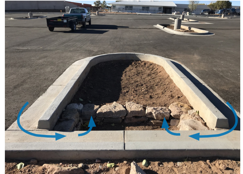
Curb Cut Inlet.
