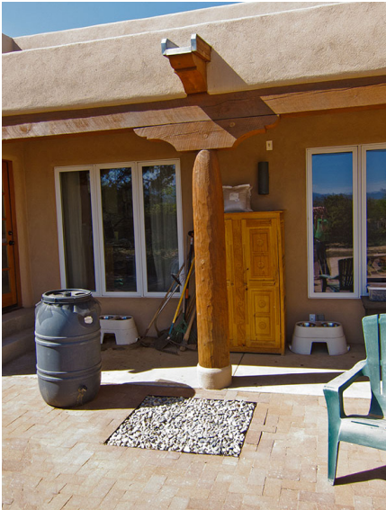
Flat roof to catchbasin.
