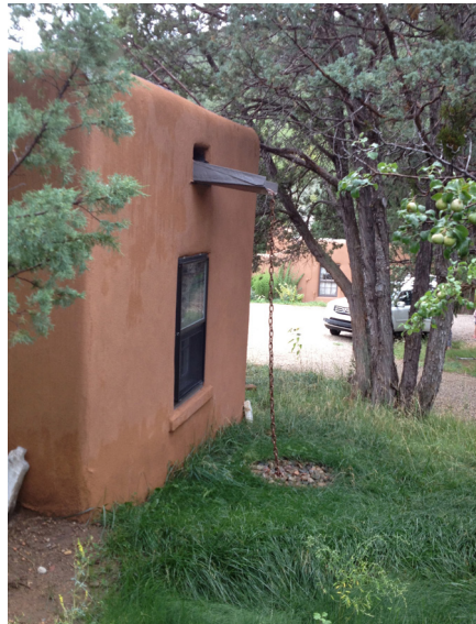
Flat roof to catchbasin with rainchain.
