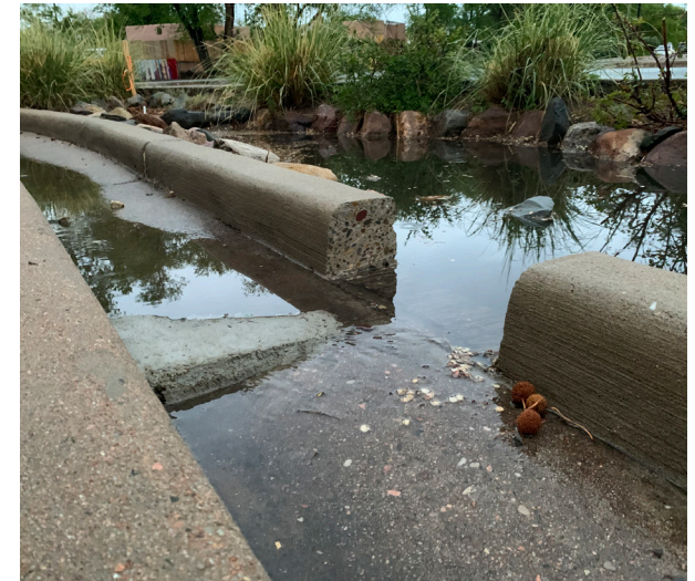
Figure 12. Covering a drain can help “daylight” stormwater so that it continues to flow above ground (instead of a darkened, below ground pipe) to a point of catchment. An estimate of increased discharge should be considered before installing a drain cap to ensure that daylighted runoff will not cause flooding, erosion, or other problems prior to reaching a GSI feature where stormwater is intended to be captured.
