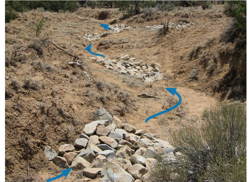
Series of One Rock Dams at Crossover Points in Channel During Installation.
