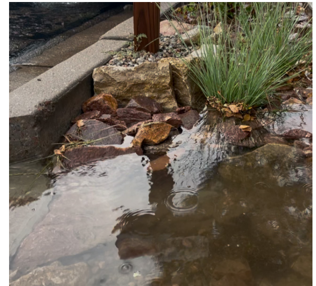
Water filling sediment trap before traveling through rain garden.
