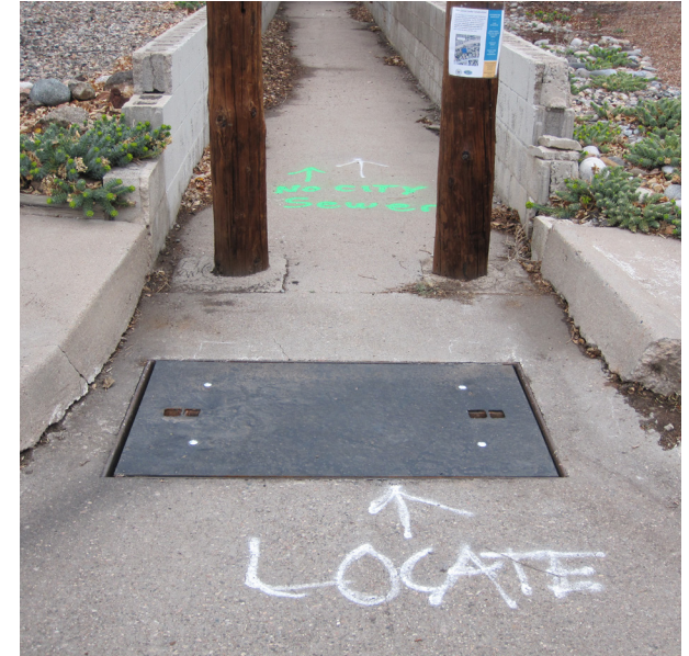
Figure 12. Covering a drain can help “daylight” stormwater so that it continues to flow above ground (instead of a darkened, below ground pipe) to a point of catchment. An estimate of increased discharge should be considered before installing a drain cap to ensure that daylighted runoff will not cause flooding, erosion, or other problems prior to reaching a GSI feature where stormwater is intended to be captured.
