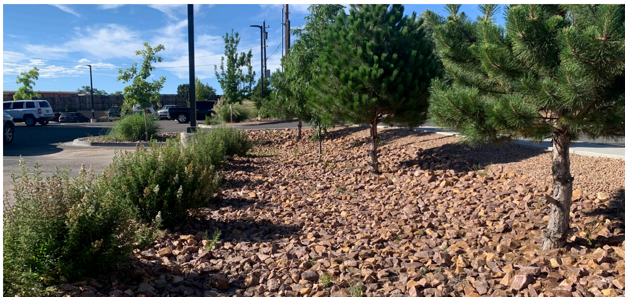
Bioswale with stone-lined channel bottom and edges (due to steep edge and bottom slope).
