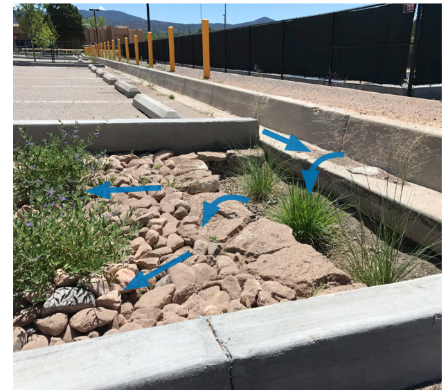
Figure 18. Examples of flow (blue arrows) into sediment traps, and approximate pooling depths before overflow into basins. Left: A small sediment trap approximately 6sqft and five inches deep will capture soil, trash, and other materials from the adjacent parking spaces. Middle: Stormwater runoff from a street is drawn into a sediment trap with a pipe overflow slightly below the elevation of the gutter. Runoff will slow, pool, and drop sediment around the pipe before stormwater overflows into the pipe and passes under the sidewalk into a bioretention basin. Right: A sediment trap in a parking space retrofitted as a rain garden. Bunch grasses in the trap help dissuade pedestrians from stepping into the area when turbid water obscures the depth. Note that while the trap on the right has a smaller volume than the middle trap, the area of runoff is \sim 1/6 the size meaning that the frequency of maintenance could be less.
