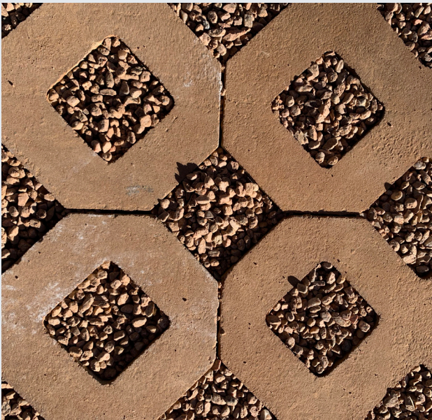
Figure 8. Concrete grid paver (left), permeable interlocking pavers (right), and plastic reinforcing grids are three forms of permeable pavers that include porous gaps to increase infiltration of stormwater to porous substrates.
