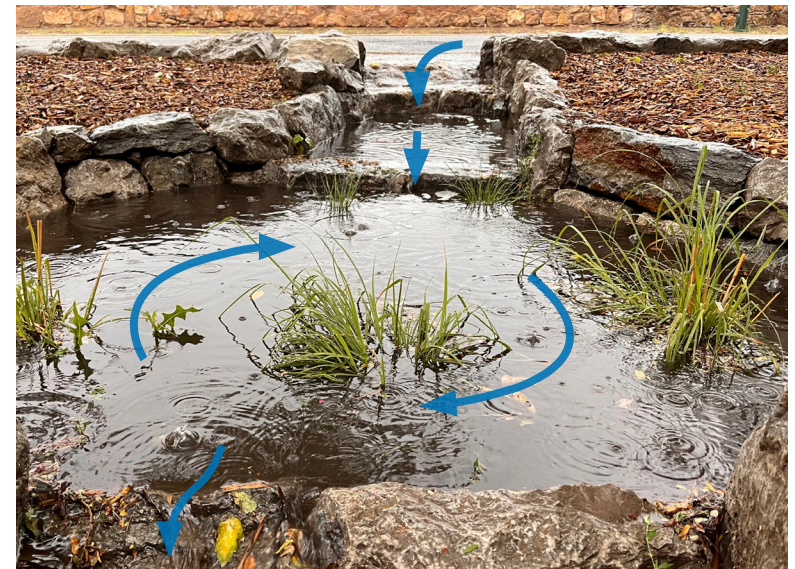
Tiered sediment trap showing pooling and filtration stages as stormwater enters GSI feature for treatment.
