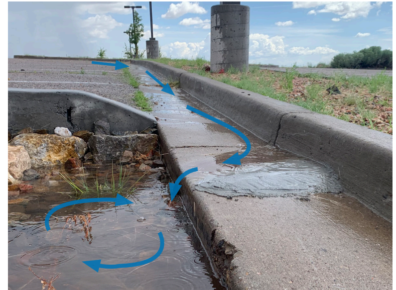
Cement Deflector Directing Stormwater Runoff into Parking Space Retrofit.
