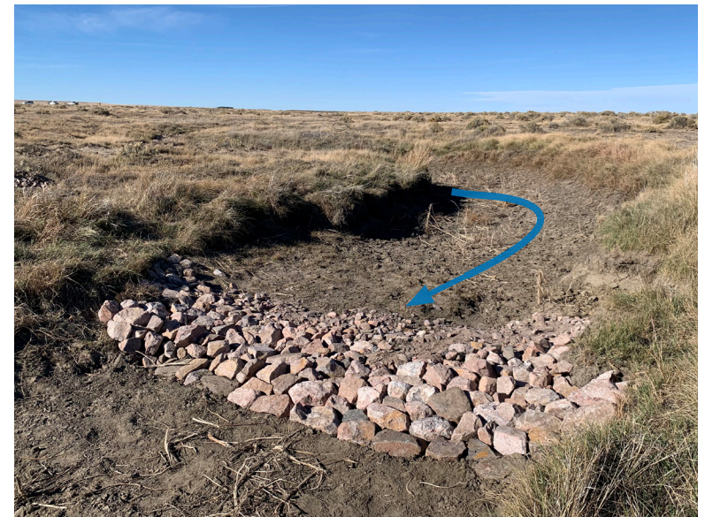
One Rock Dam at Channel Crossover.
