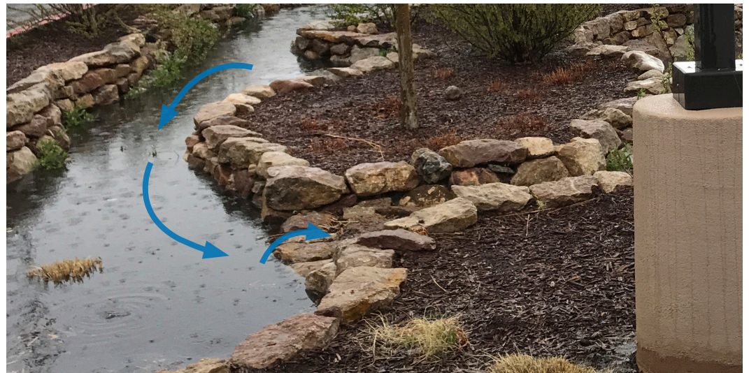
Figure 19. An example of a weir (blue arrows) in a rain garden which forces stormwater to pool a certain depth before it can overflow to the next basin. Weirs can concentrate stormwater near trees to enhance irrigation, above woodchip sponges to improve filtration, or simply to slow stormwater velocity as it passes through a GSI feature.
