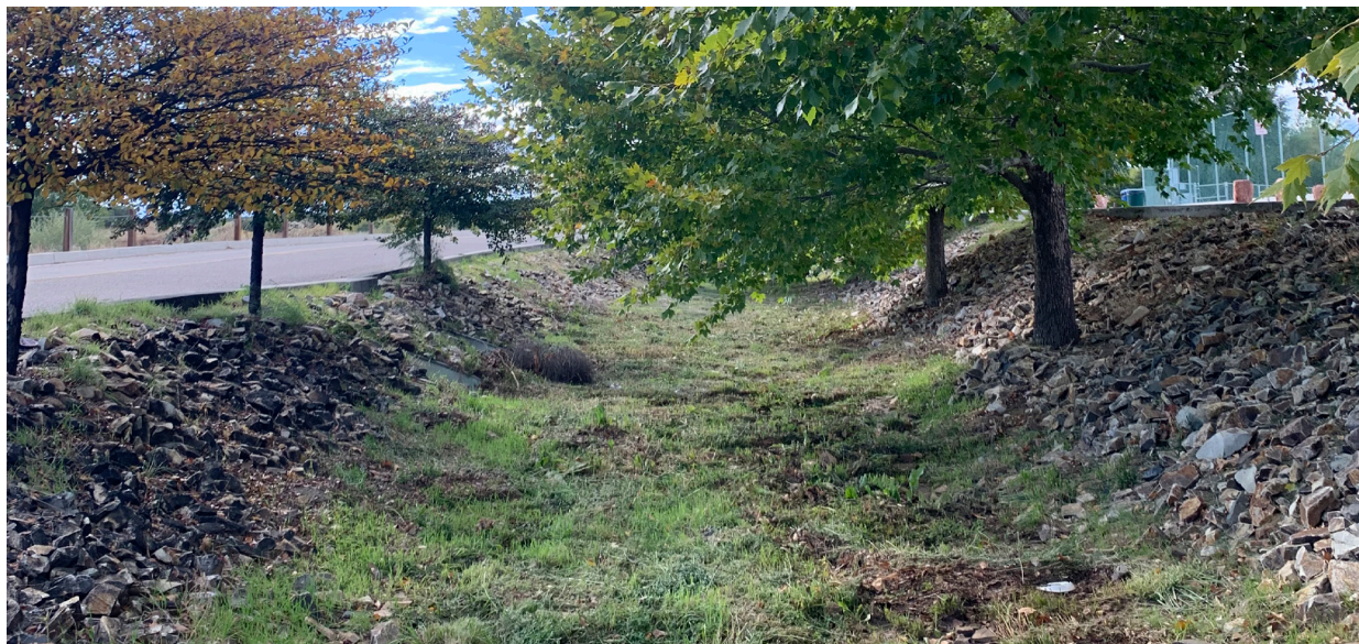
Bioswale with cobble edges (due to steep edge slope) and seeded grass bottom (due to gradual bottom slope).
