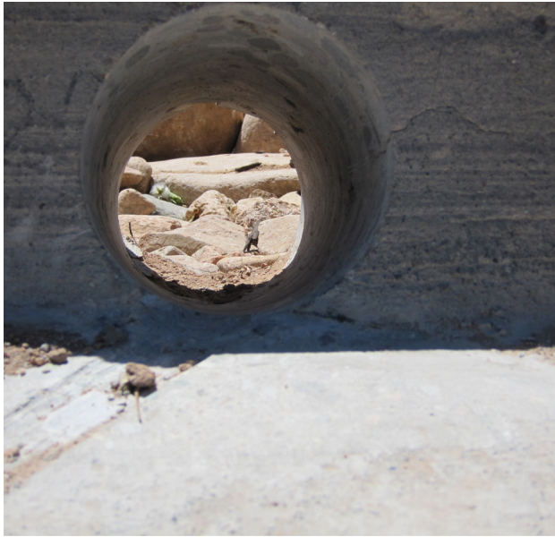
Figure 14. Curb cores (left) maintain the integrity of a curb, but are more prone to plugging with sediment and therefore not generally recommended. Flush curbs (middle) can maximize inflow, but fail to concentrate sediment at a point where it can be managed. Flush curbs might also necessitate the introduction of boulders or vertical core-filled metal pipes to prevent vehicles from damaging vegetation/soil. Moderate (18-24 inches wide) curb openings (right) are ideal for concentrating catchment at a defined point where sediment traps can be installed.
