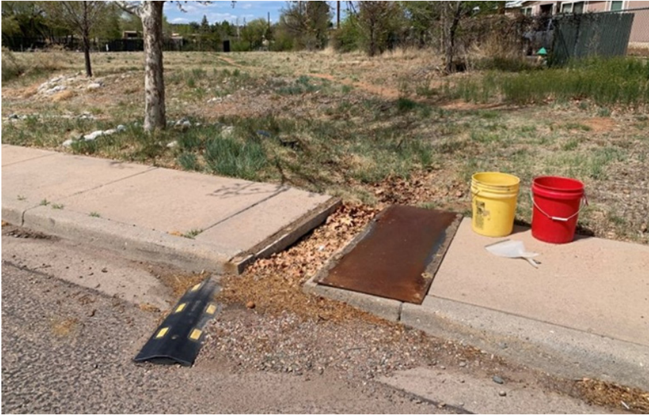
Sediment and debris built up at the inlet of a GSI feature due to lack of maintenance.
