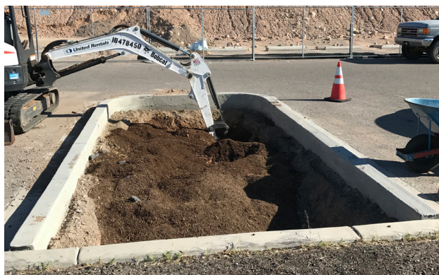
Figure 22. Bio-retention basins (opposite page) often include deep layers or mixes of woodchips, compost, sand, and gravel to infiltrate and filter large volumes of stormwater runoff. The image includes 12-inches of woodchips that were subsequently capped with a mixture of compost and sand to rapidly infiltrate and filter runoff from over 1-acre of neighborhood streets. The compost/sand mix prevented the woodchips from floating in roughly 18-inches of potential pooling depth.
