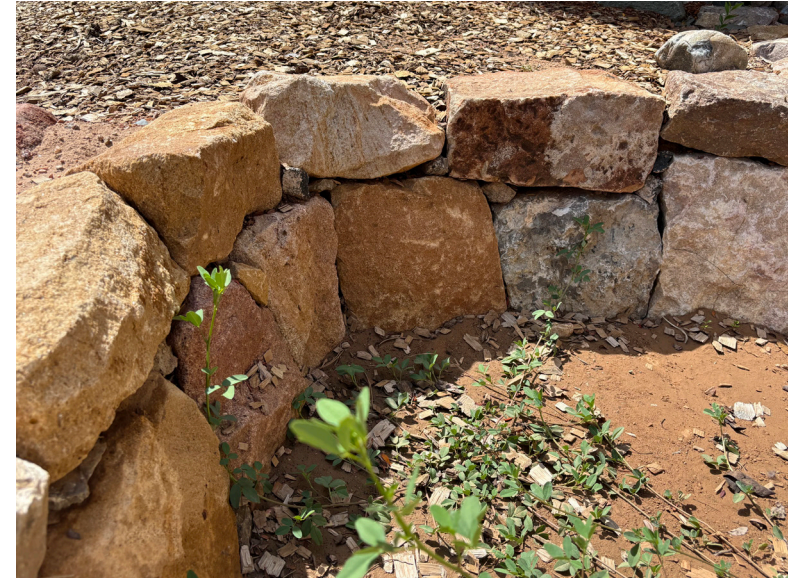
Basin border constructed with Stacked Rock.
