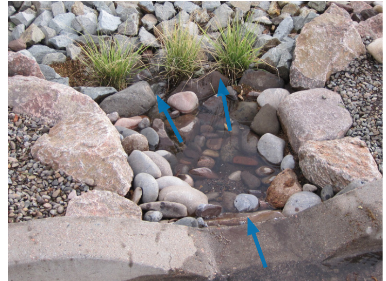
Sediment trap with float grass filter behind to block debris from entering the rest of the GSI feature.
