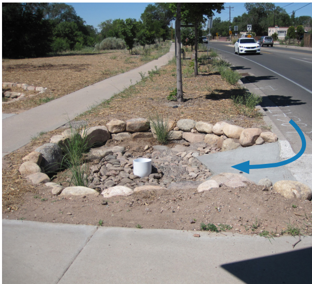
Figure 18. Examples of flow (blue arrows) into sediment traps, and approximate pooling depths before overflow into basins. Left: A small sediment trap approximately 6sqft and five inches deep will capture soil, trash, and other materials from the adjacent parking spaces. Middle: Stormwater runoff from a street is drawn into a sediment trap with a pipe overflow slightly below the elevation of the gutter. Runoff will slow, pool, and drop sediment around the pipe before stormwater overflows into the pipe and passes under the sidewalk into a bioretention basin. Right: A sediment trap in a parking space retrofitted as a rain garden. Bunch grasses in the trap help dissuade pedestrians from stepping into the area when turbid water obscures the depth. Note that while the trap on the right has a smaller volume than the middle trap, the area of runoff is \sim 1/6 the size meaning that the frequency of maintenance could be less.
