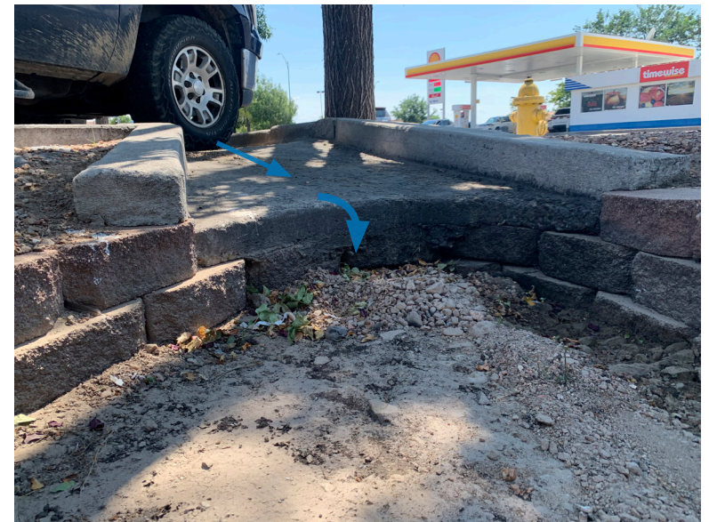
Curb Cut Inlet with Armored Sides.
