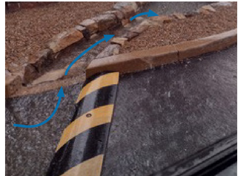
Speed Bump Deflector In Rain Directing Stormwater Runoff into Curbside Rain Garden.
