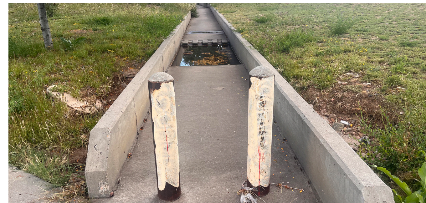
Storm drain cap in concrete channel.
