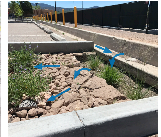
Figure 18. Examples of flow (blue arrows) into sediment traps, and approximate pooling depths before overflow into basins. Left: A small sediment trap approximately 6sqft and five inches deep will capture soil, trash, and other materials from the adjacent parking spaces. Middle: Stormwater runoff from a street is drawn into a sediment trap with a pipe overflow slightly below the elevation of the gutter. Runoff will slow, pool, and drop sediment around the pipe before stormwater overflows into the pipe and passes under the sidewalk into a bioretention basin. Right: A sediment trap in a parking space retrofitted as a rain garden. Bunch grasses in the trap help dissuade pedestrians from stepping into the area when turbid water obscures the depth. Note that while the trap on the right has a smaller volume than the middle trap, the area of runoff is ~1/6 the size meaning that the frequency of maintenance could be less.
