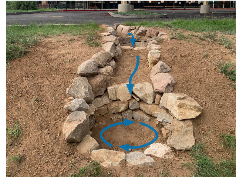
Zuni Bowl Under Construction.
