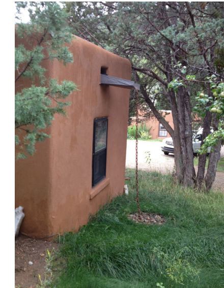
Flat roof to catchbasin with rainchain.
