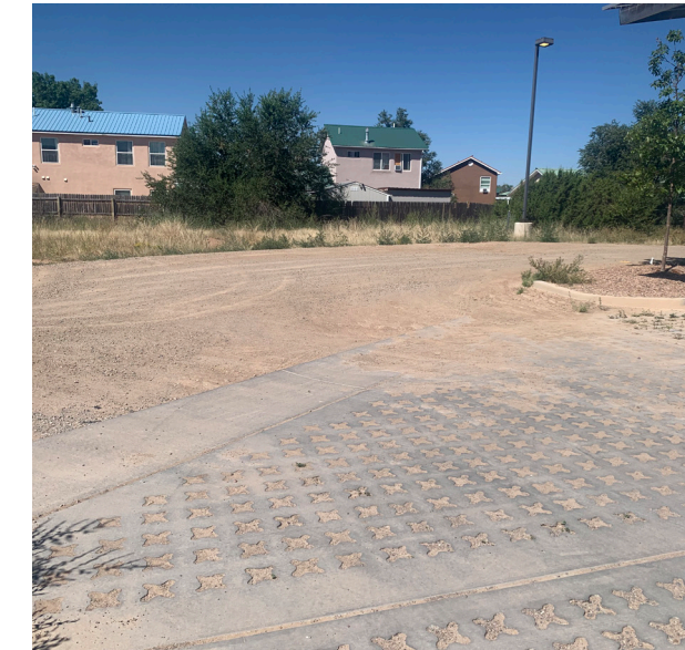
Figure 9. Examples of how unmaintained permeable pavers can lose infiltration capacity due to fine textures plugging the porous gaps (left and middle) which results in standing water on the surface (right).
