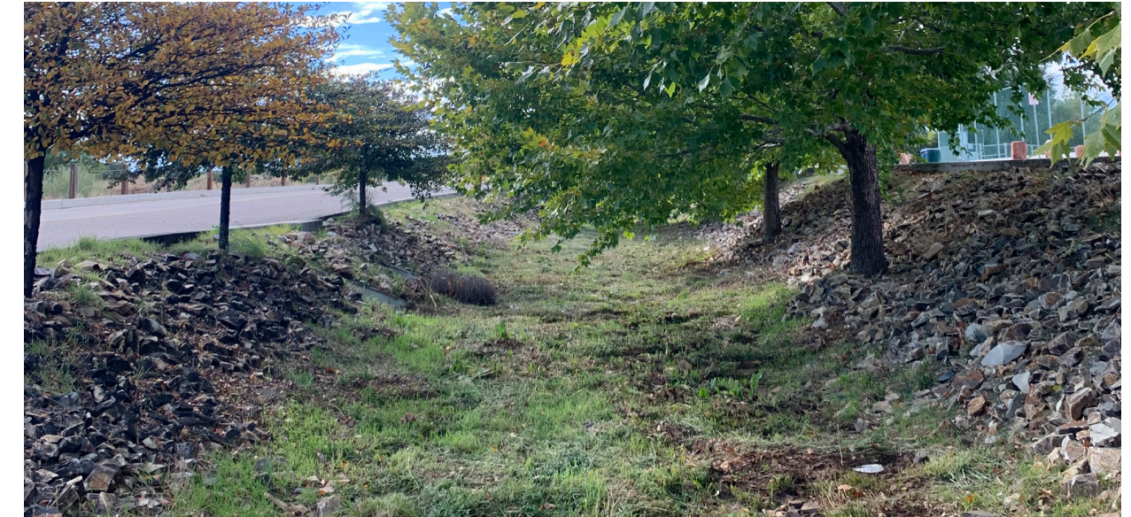
Bioswale with cobble edges (due to steep edge slope) and seeded grass bottom (due to gradual bottom slope).
