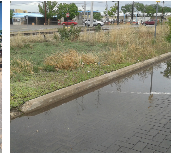
Figure 9. Examples of how unmaintained permeable pavers can lose infiltration capacity due to fine textures plugging the porous gaps (left and middle) which results in standing water on the surface (right).
