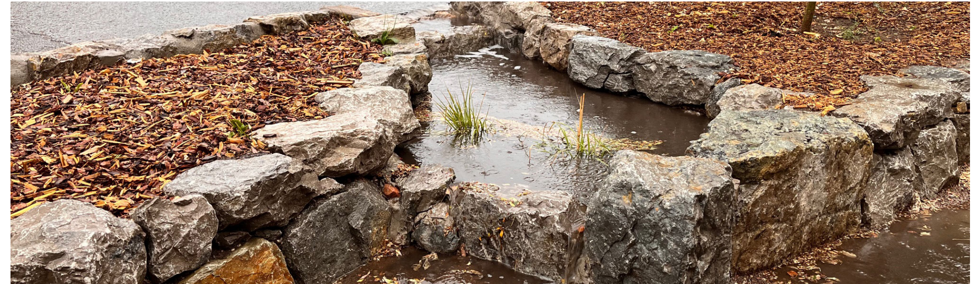
Water filling and pooling in sediment trap before traveling through rain garden.
