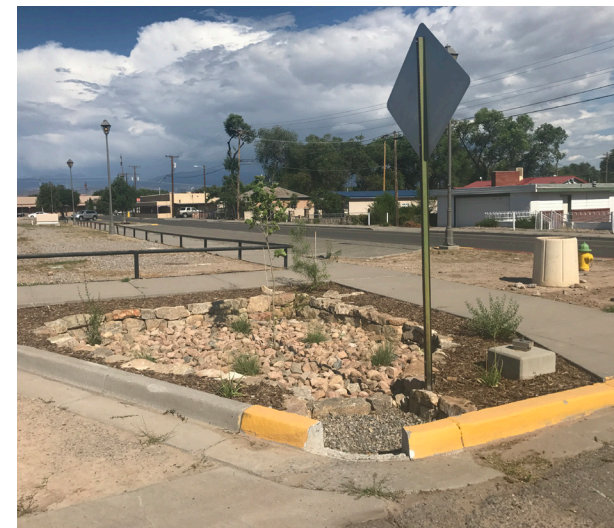
Figure 15. The width of a stormwater inlet for comparable areas of runoff might vary depending on the direction of flow at the capture point. If stormwater is running perpendicular to flow (left), then a smaller opening might suffice. If stormwater is running parallel to the inlet and must make a 90 degree turn into the basin from a small area of runoff (middle), then the inlet width could be improved with a small deflector. As the area of runoff increases, if stormwater is running parallel to the inlet, then a much wider inlet with steeper slope might be required (right). Note that during high intensity storms, runoff in the photo to the right can still bypass the inlet due to originating from approximately 20,000sqft of asphalt area.
