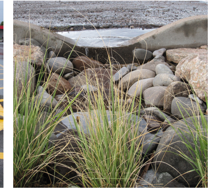
Figure 14. Curb cores (left) maintain the integrity of a curb, but are more prone to plugging with sediment and therefore not generally recommended. Flush curbs (middle) can maximize inflow, but fail to concentrate sediment at a point where it can be managed. Flush curbs might also necessitate the introduction of boulders or vertical core-filled metal pipes to prevent vehicles from damaging vegetation/soil. Moderate (18-24 inches wide) curb openings (right) are ideal for concentrating catchment at a defined point where sediment traps can be installed.
