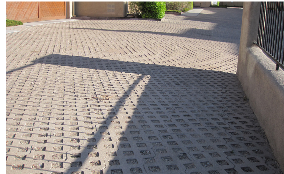
Figure 10. Example of concrete grid paver driveway with minimal sediment sources (left) and permeable interlocking pavers with curb cuts (right) which could direct excess stormwater into other GSI features such as rain gardens (not shown).
