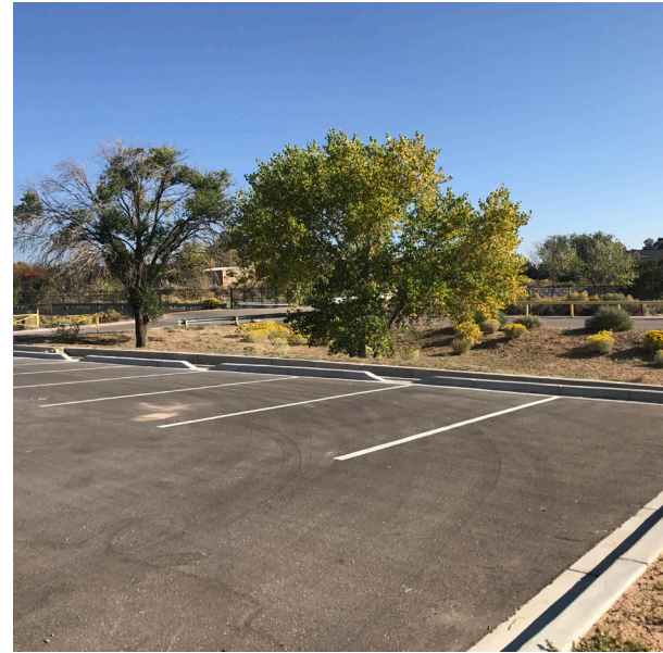
Figure 13. Numerous curb inlets along a median edge might promote better stormwater catchment than a singular opening. Extra curb cut openings are good where maximizing inflow is desired, where unevenness of gutter or adjacent impervious areas might require multiple inlets, or to prevent pooling water on parking areas if the curb is on contour (i.e. minimal slope).captured.
