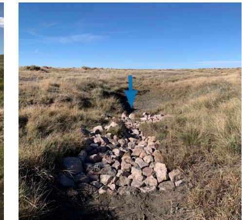
Figure 6. Left to right: A media luna (photo courtesy of Minesh Bacrania), one rock dam, Zuni bowl, and rock rundown are structures used to mitigate stormwater runoff and erosion at low energy upland sites.
