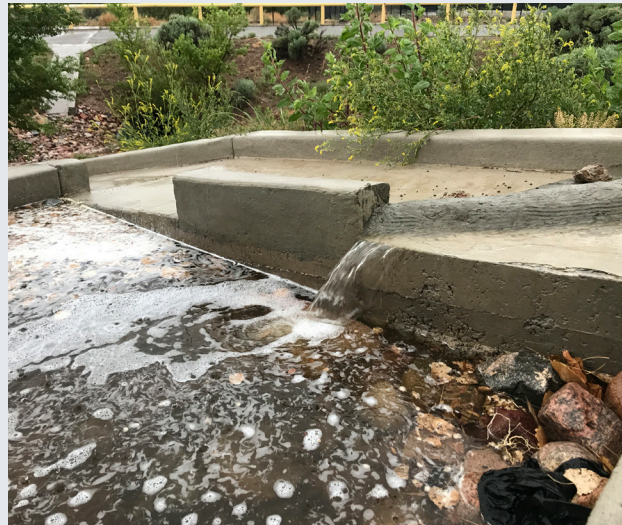
Figure 11. Examples of cement gutter (left and right) and asphalt speed bump deflectors redirecting stormwater into rain garden inlets.
