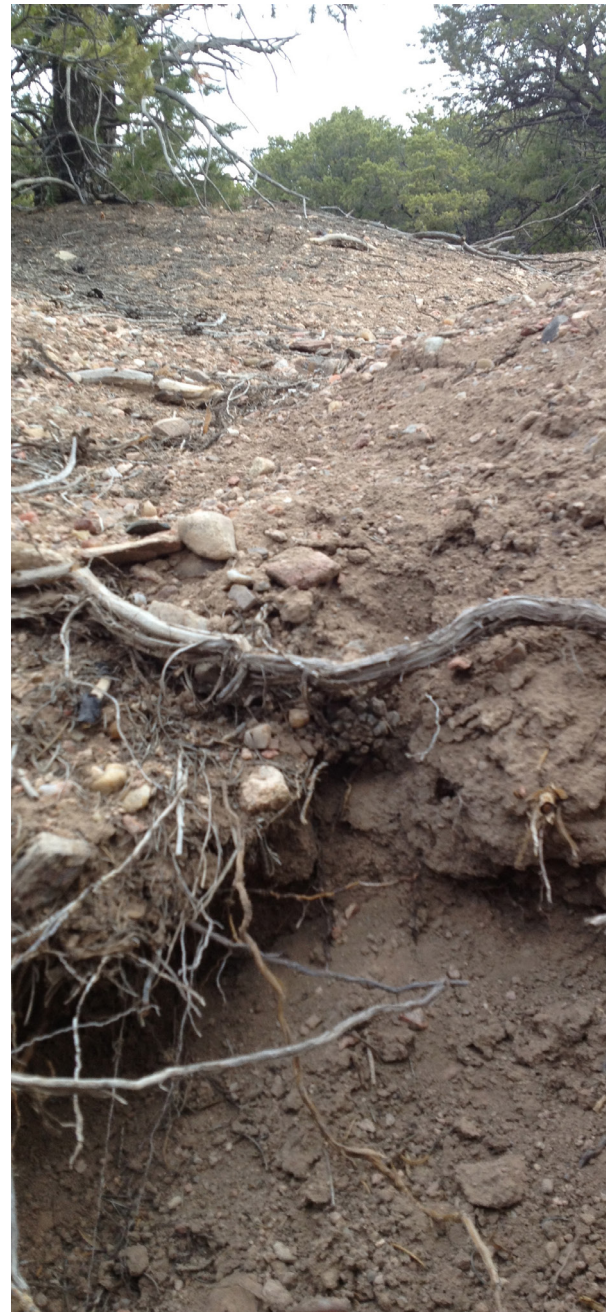
A headcut (foreground); eroding upslope, compromising topsoil and tree roots.
