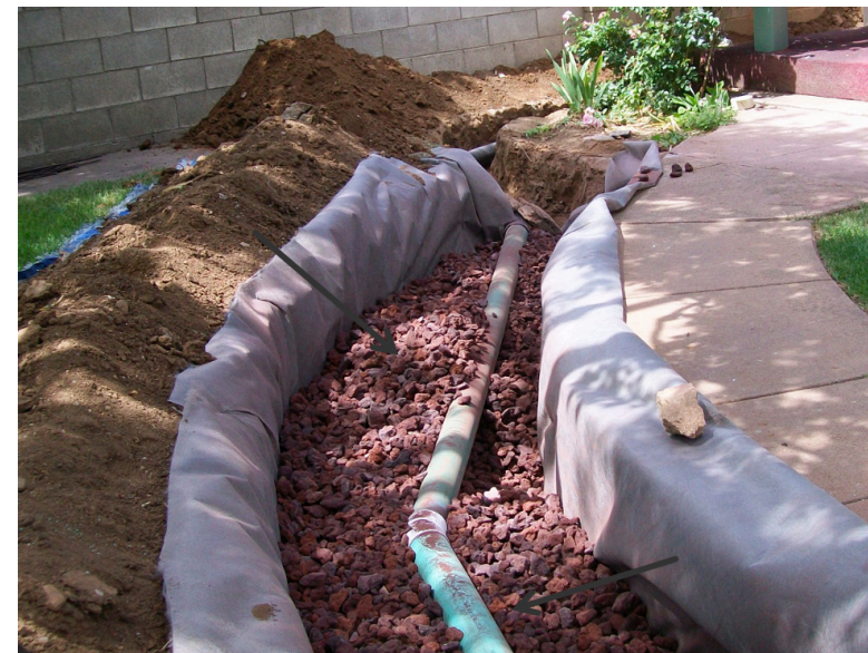
Pumice wick trench, lined with geotextile fabric and filled.
