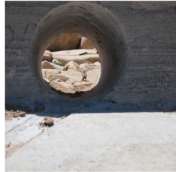
Figure 14. Curb cores (left) maintain the integrity of a curb, but are more prone to plugging with sediment and therefore not generally recommended. Flush curbs (middle) can maximize inflow, but fail to concentrate sediment at a point where it can be managed. Flush curbs might also necessitate the introduction of boulders or vertical core-filled metal pipes to prevent vehicles from damaging vegetation/soil. Moderate (18-24 inches wide) curb openings (right) are ideal for concentrating catchment at a defined point where sediment traps can be installed.
