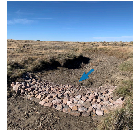
Figure 6. Left to right: A media luna (photo courtesy of Minesh Bacrania), one rock dam, Zuni bowl, and rock rundown are structures used to mitigate stormwater runoff and erosion at low energy upland sites.
