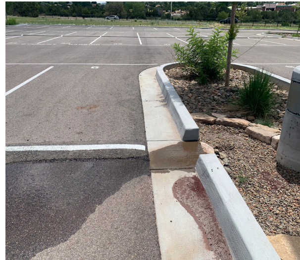
Figure 11. Examples of cement gutter (left and right) and asphalt speed bump deflectors redirecting stormwater into rain garden inlets.
