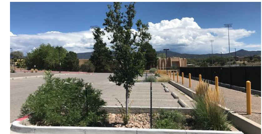
From left to right: Parking space retrofit rain garden at varying stages of construction.
