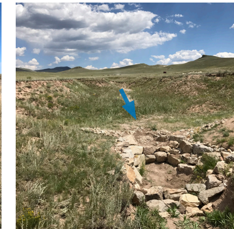
Figure 6. Left to right: A media luna (photo courtesy of Minesh Bacrania), one rock dam, Zuni bowl, and rock rundown are structures used to mitigate stormwater runoff and erosion at low energy upland sites.
