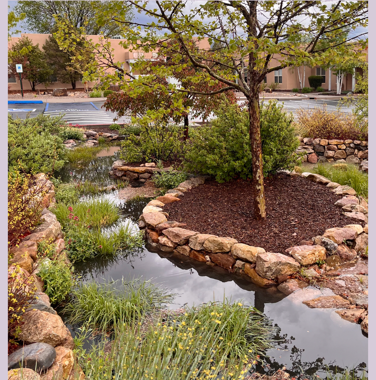
Slow movement of springtime stormwater through native grasses in GSI feature.
