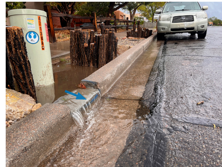
Curb cut outlet at lowest point.
