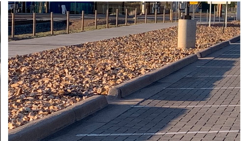
Figure 10. Example of concrete grid paver driveway with minimal sediment sources (left) and permeable interlocking pavers with curb cuts (right) which could direct excess stormwater into other GSI features such as rain gardens (not shown).
