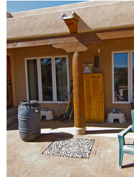
Flat roof to catchbasin.
