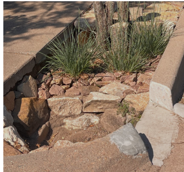
Sediment trap with float grass filter behind to block debris from entering the rest of the GSI feature, dry.
