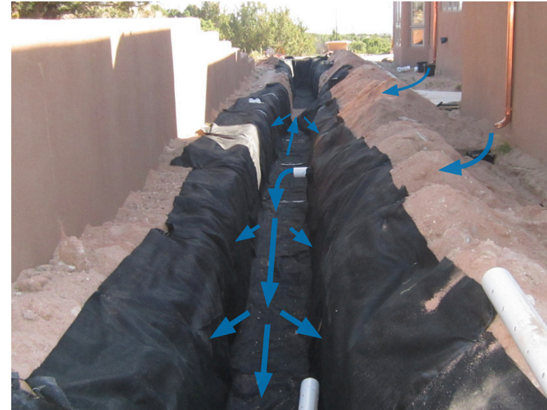
Pumice wick trench, lined with geotextile fabric and unfilled.
