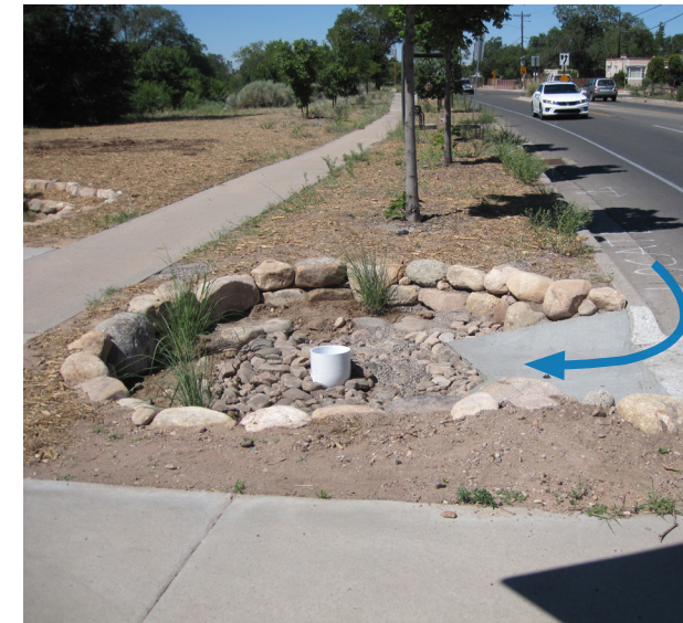
Figure 18. Examples of flow (blue arrows) into sediment traps, and approximate pooling depths before overflow into basins. Left: A small sediment trap approximately 6sqft and five inches deep will capture soil, trash, and other materials from the adjacent parking spaces. Middle: Stormwater runoff from a street is drawn into a sediment trap with a pipe overflow slightly below the elevation of the gutter. Runoff will slow, pool, and drop sediment around the pipe before stormwater overflows into the pipe and passes under the sidewalk into a bioretention basin. Right: A sediment trap in a parking space retrofitted as a rain garden. Bunch grasses in the trap help dissuade pedestrians from stepping into the area when turbid water obscures the depth. Note that while the trap on the right has a smaller volume than the middle trap, the area of runoff is ~1/6 the size meaning that the frequency of maintenance could be less.
