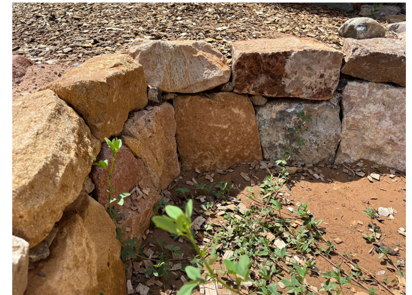
Basin border constructed with Stacked Rock.
