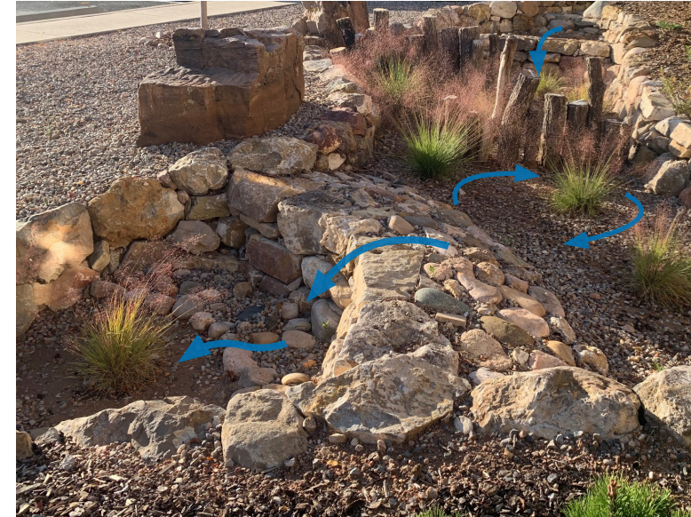
Stone weir construction.
