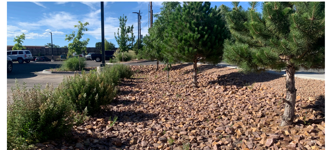
Bioswale with stone-lined channel bottom and edges (due to steep edge and bottom slope).
