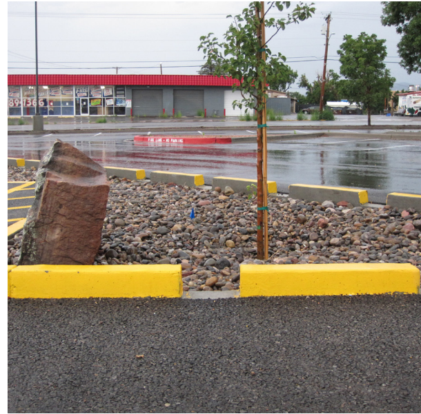
Figure 13. Numerous curb inlets along a median edge might promote better stormwater catchment than a singular opening. Extra curb cut openings are good where maximizing inflow is desired, where unevenness of gutter or adjacent impervious areas might require multiple inlets, or to prevent pooling water on parking areas if the curb is on contour (i.e. minimal slope).captured.
