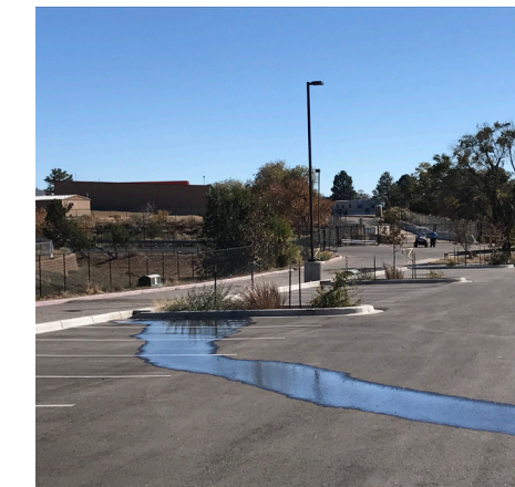
Figure 5. The rain garden on the left maximizes stormwater catchment because asphalt grades were installed properly. The rain garden on the right misses almost 2,000sqft of runoff (i.e. thousands of gallons annually) because asphalt grades were off by an inch!
