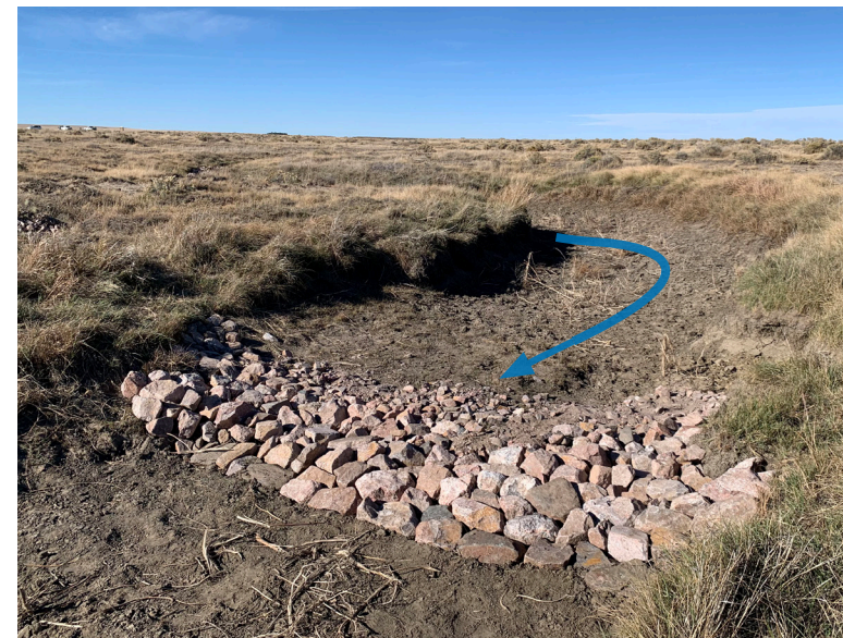
One Rock Dam at Channel Crossover.
