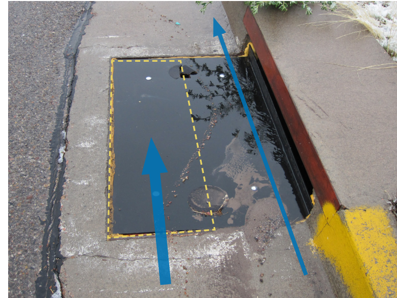
Drain cap showing how the omission of half its possible area (i.e. yellow dotted line) would redirect flow during smaller storm events, but drain larger runoff events.
