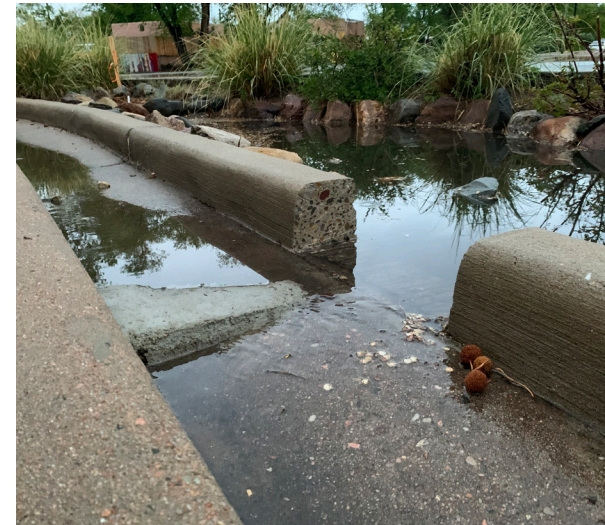
Figure 12. Covering a drain can help “daylight” stormwater so that it continues to flow above ground (instead of a darkened, below ground pipe) to a point of catchment. An estimate of increased discharge should be considered before installing a drain cap to ensure that daylighted runoff will not cause flooding, erosion, or other problems prior to reaching a GSI feature where stormwater is intended to be captured.
