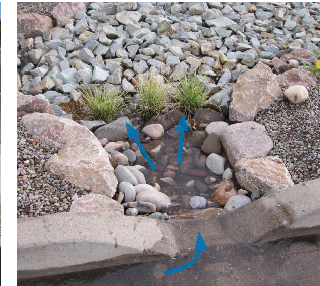
Figure 18. Examples of flow (blue arrows) into sediment traps, and approximate pooling depths before overflow into basins. Left: A small sediment trap approximately 6sqft and five inches deep will capture soil, trash, and other materials from the adjacent parking spaces. Middle: Stormwater runoff from a street is drawn into a sediment trap with a pipe overflow slightly below the elevation of the gutter. Runoff will slow, pool, and drop sediment around the pipe before stormwater overflows into the pipe and passes under the sidewalk into a bioretention basin. Right: A sediment trap in a parking space retrofitted as a rain garden. Bunch grasses in the trap help dissuade pedestrians from stepping into the area when turbid water obscures the depth. Note that while the trap on the right has a smaller volume than the middle trap, the area of runoff is ~1/6 the size meaning that the frequency of maintenance could be less.
