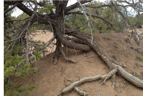
Large pinon tree roots exposed on hillside due to erosion from weathering and lack of vegetation
