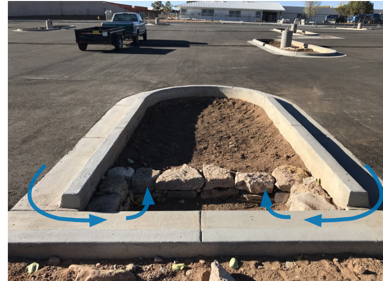
Curb Cut Inlet.
