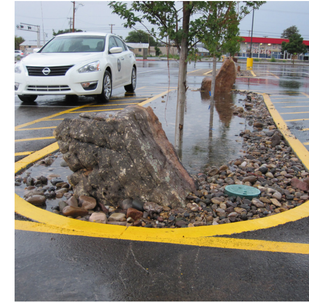
Figure 14. Curb cores (left) maintain the integrity of a curb, but are more prone to plugging with sediment and therefore not generally recommended. Flush curbs (middle) can maximize inflow, but fail to concentrate sediment at a point where it can be managed. Flush curbs might also necessitate the introduction of boulders or vertical core-filled metal pipes to prevent vehicles from damaging vegetation/soil. Moderate (18-24 inches wide) curb openings (right) are ideal for concentrating catchment at a defined point where sediment traps can be installed.
