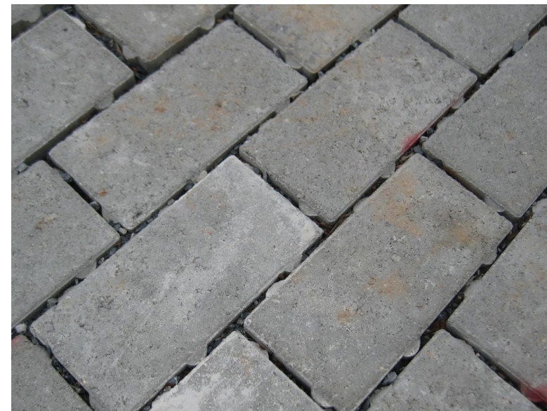
Permeable Interlocking Concrete Pavers (PICP) (Image Credit: Homeguide.com) In ideal style for Southwestern regions. Staggered ridges in between gaps prevent shifting that may block openings. Wider [than standard] gaps increase filtration potential and mitigate sediment build up in arid climates.
