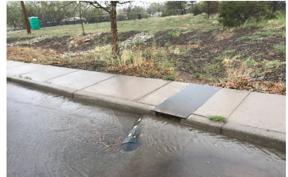
Consequence of sediment and debris build up: water cannot enter GSI feature.
