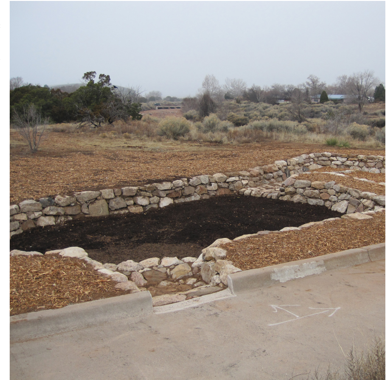
Bioretention Basin with Stone Edges Prior to Planting
