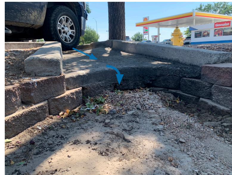
Curb Cut Inlet with Armored Sides.
