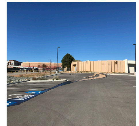
Figure 5. The rain garden on the left maximizes stormwater catchment because asphalt grades were installed properly. The rain garden on the right misses almost 2,000sqft of runoff (i.e. thousands of gallons annually) because asphalt grades were off by an inch!
