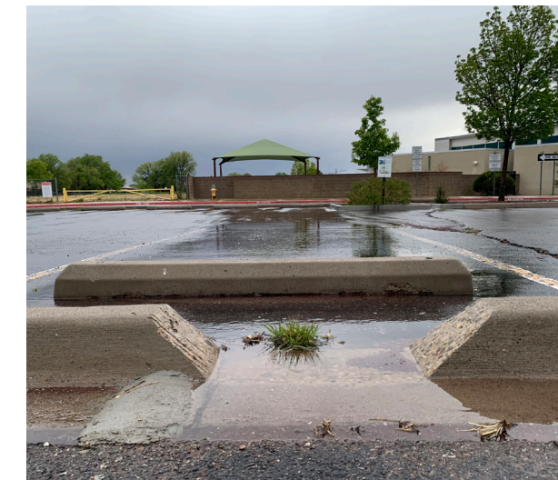
Figure 15. The width of a stormwater inlet for comparable areas of runoff might vary depending on the direction of flow at the capture point. If stormwater is running perpendicular to flow (left), then a smaller opening might suffice. If stormwater is running parallel to the inlet and must make a 90 degree turn into the basin from a small area of runoff (middle), then the inlet width could be improved with a small deflector. As the area of runoff increases, if stormwater is running parallel to the inlet, then a much wider inlet with steeper slope might be required (right). Note that during high intensity storms, runoff in the photo to the right can still bypass the inlet due to originating from approximately 20,000sqft of asphalt area.
