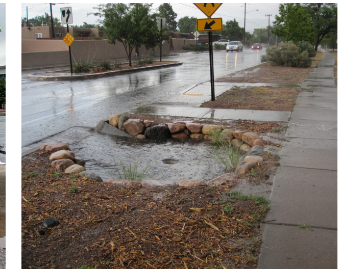
Figure 15. The width of a stormwater inlet for comparable areas of runoff might vary depending on the direction of flow at the capture point. If stormwater is running perpendicular to flow (left), then a smaller opening might suffice. If stormwater is running parallel to the inlet and must make a 90 degree turn into the basin from a small area of runoff (middle), then the inlet width could be improved with a small deflector. As the area of runoff increases, if stormwater is running parallel to the inlet, then a much wider inlet with steeper slope might be required (right). Note that during high intensity storms, runoff in the photo to the right can still bypass the inlet due to originating from approximately 20,000sqft of asphalt area.
