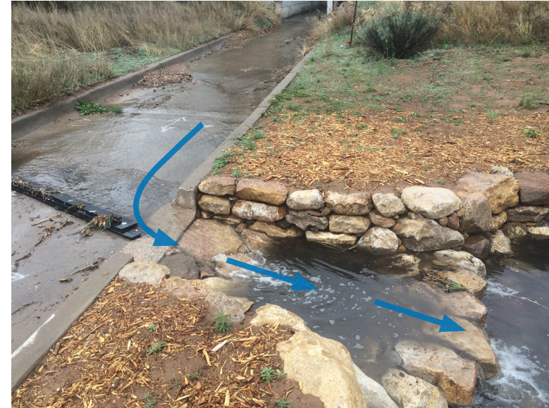
Curb Cut Inlet with Deflector.
