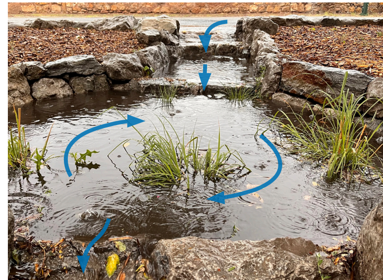
Tiered sediment trap showing pooling and filtration stages as stormwater enters GSI feature for treatment.
