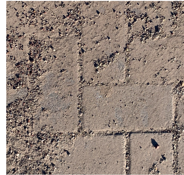
Figure 9. Examples of how unmaintained permeable pavers can lose infiltration capacity due to fine textures plugging the porous gaps (left and middle) which results in standing water on the surface (right).
