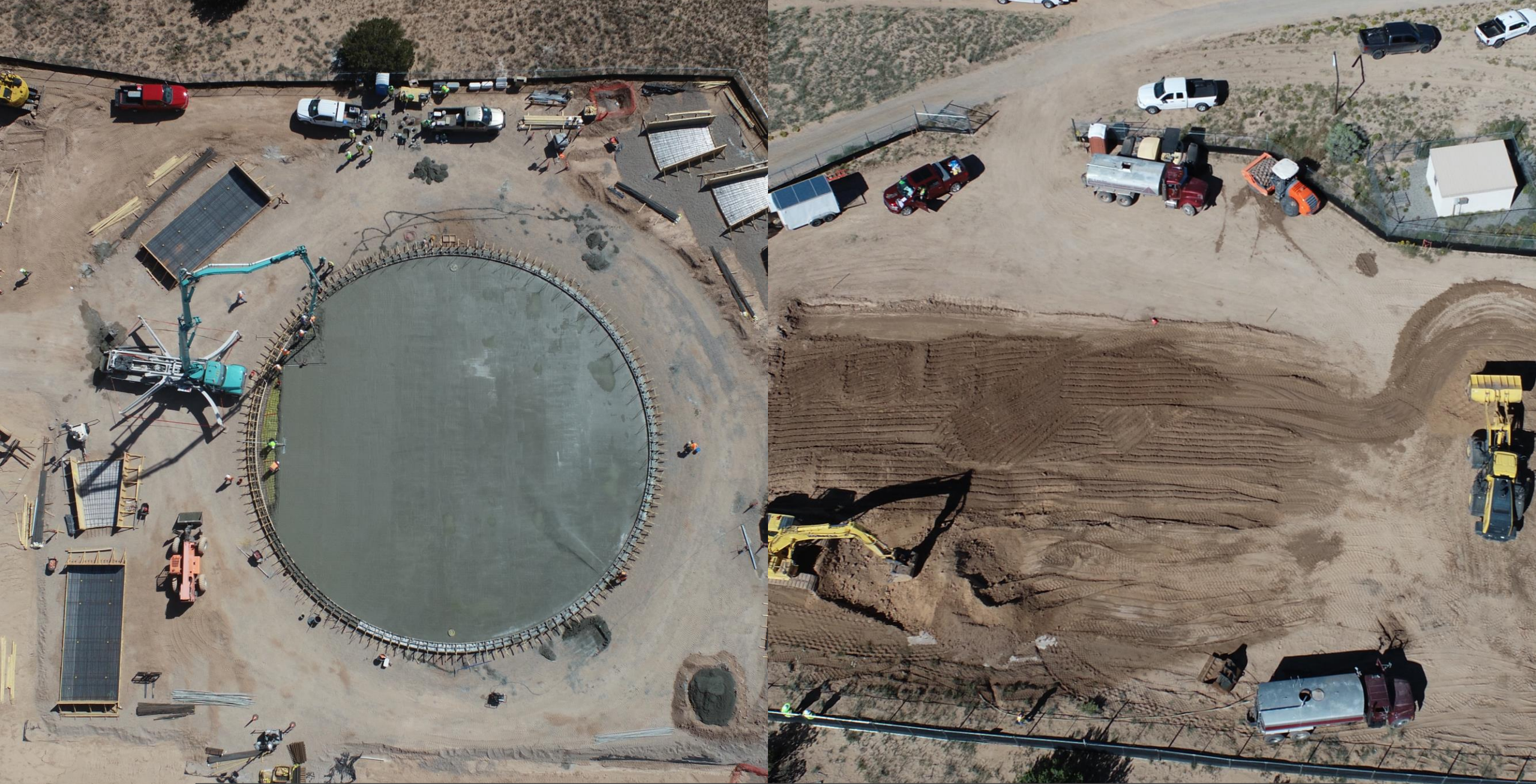
PBRWS - TANK CONSTRUCTION POJOAQUE PUEBLO
