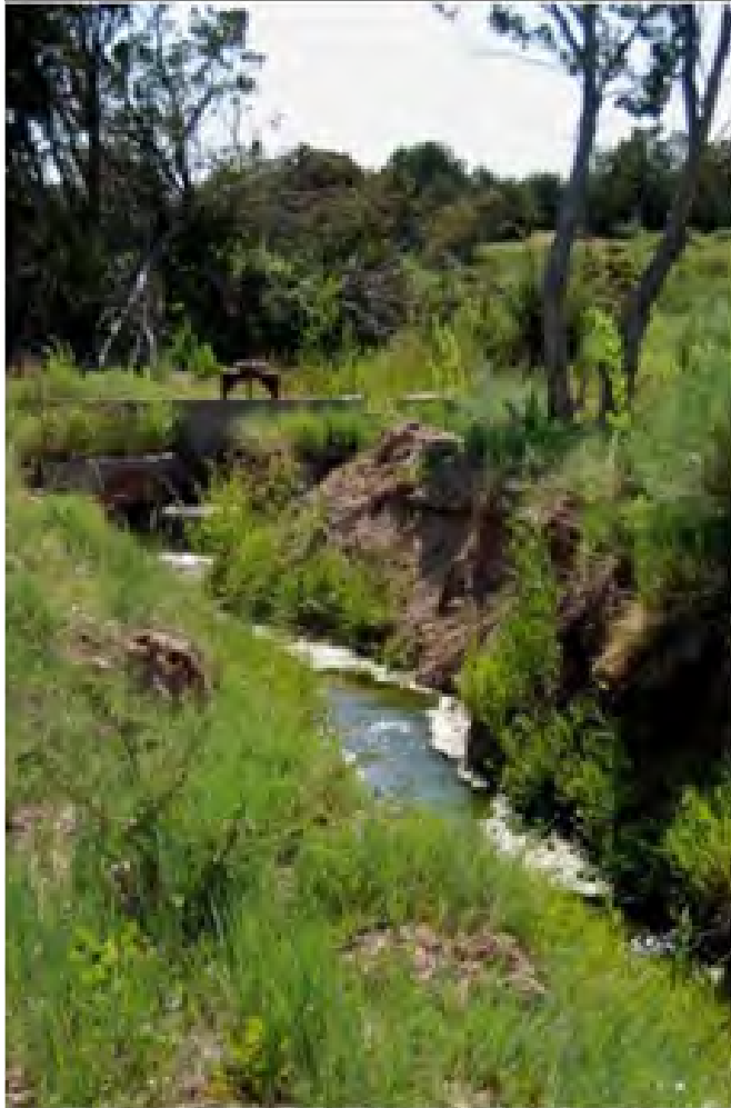
Acequia La Cienega Diversion Headgate, Photo circa 2015.
