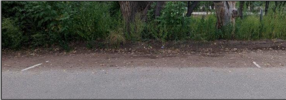
Figure 40: Marked parking spaces on Bishops Lodge Road
