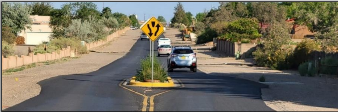
Figure 24: Median Island on Meadowlark Lane
