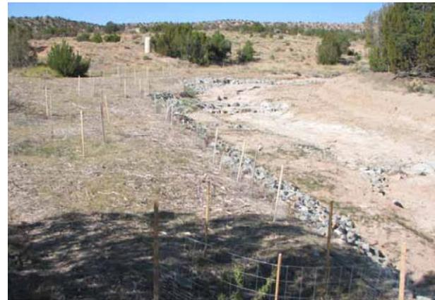
**Figure 7a.** (Left): Example of an entrenched meander channel that undermined and dewatered a wetland upstream of the Arroyo de los Angeles in the Galisteo Basin (viewing upstream).
