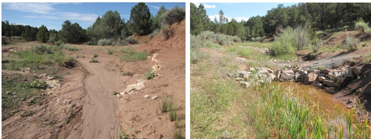
**Figure 9a.** (Left): A series of rock cross vanes in Cañoncito Arroyo (Eldorado Community Preserve) wetlands raised the grade of the stream and made point bars, the floodplain and adjacent riverine wetlands accessible to lower level (more frequent) floods.
