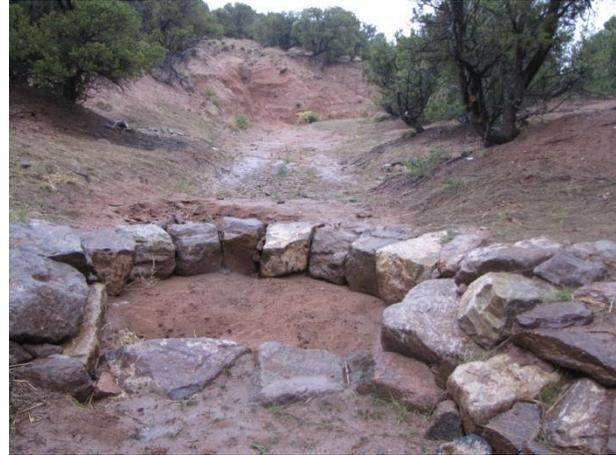
**Figure 10a.** (Left): One-Rock-Dam and rock rundown in Arroyo Saiz in Santa Fe (looking upstream). Photo by Earth Works Institute 2010.
