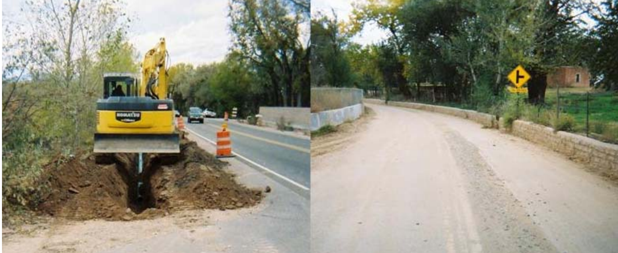
Figure 4-1 Recent IHS Pipeline Installation Parallel to NM 502 and in County Road
