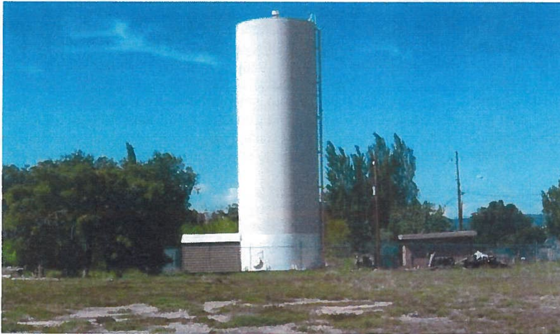
Agua Fria Community Water Association Water Tower and Well House
