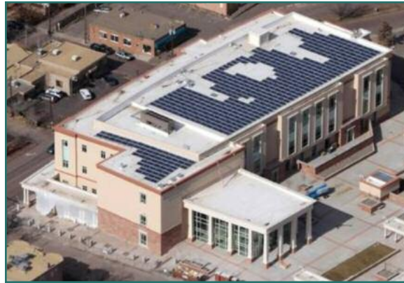
113 kilowatt solar system on the roof of the new Judicial Complex – a LEED Gold green building.” Photo Credit: Eagle’s Eye – Aerial Photo Solutions
